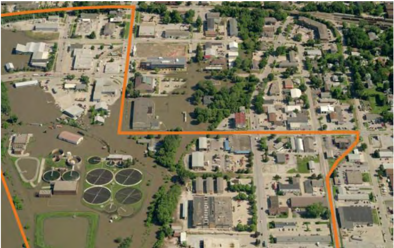
Figure 2: Flood Impacted Area
