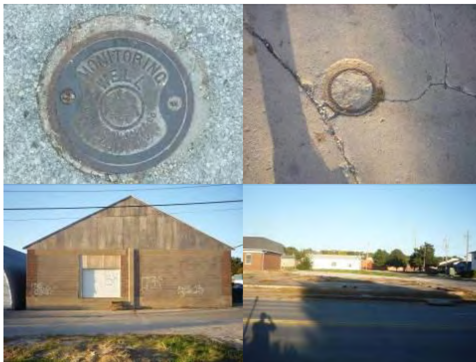
Figure 10: Examples of Site Conditions along Gilbert Street
