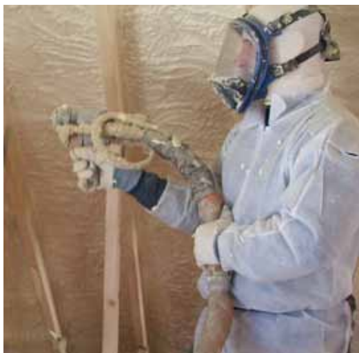
Expensive but comprehensive. Spray foam is applied as a liquid, but quickly foams and expands to fill the insulating space. Photo courtesy of Spray Tech Foam
