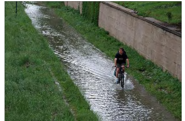
Cherry Creek bike path during flooding
