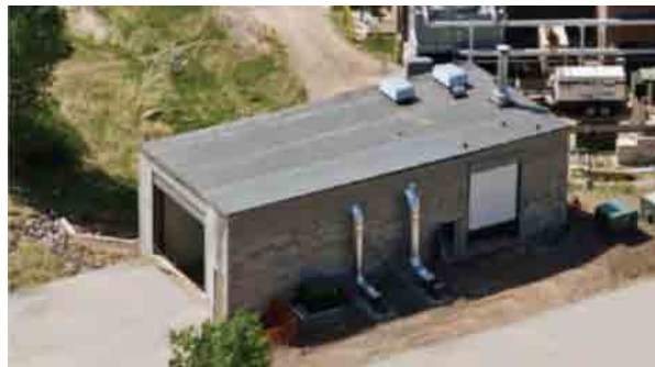
Figure 12: Central Biomass Heating Plant on the NREL Campus (Source: NREL Pix Photo Library)
