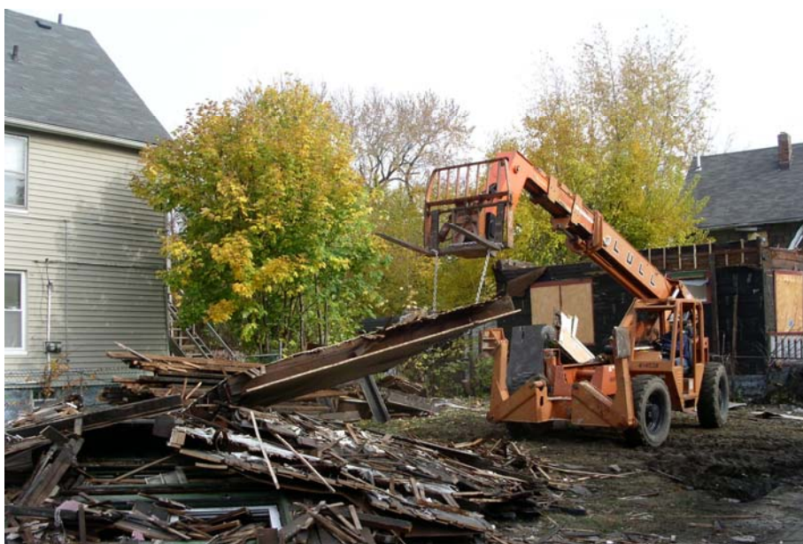
Photo 6 – Cleveland Deconstruction Initiative – Wall Panel Placement for Dismantling
