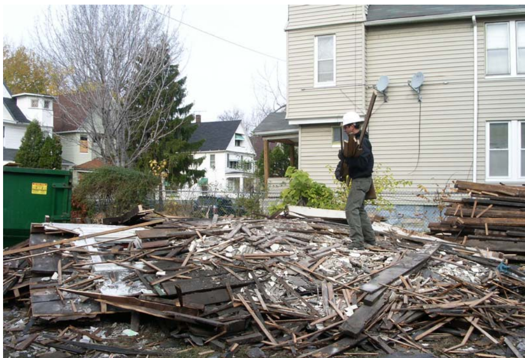
Photo 8 – Cleveland Deconstruction Initiative – Hand Dismantling
