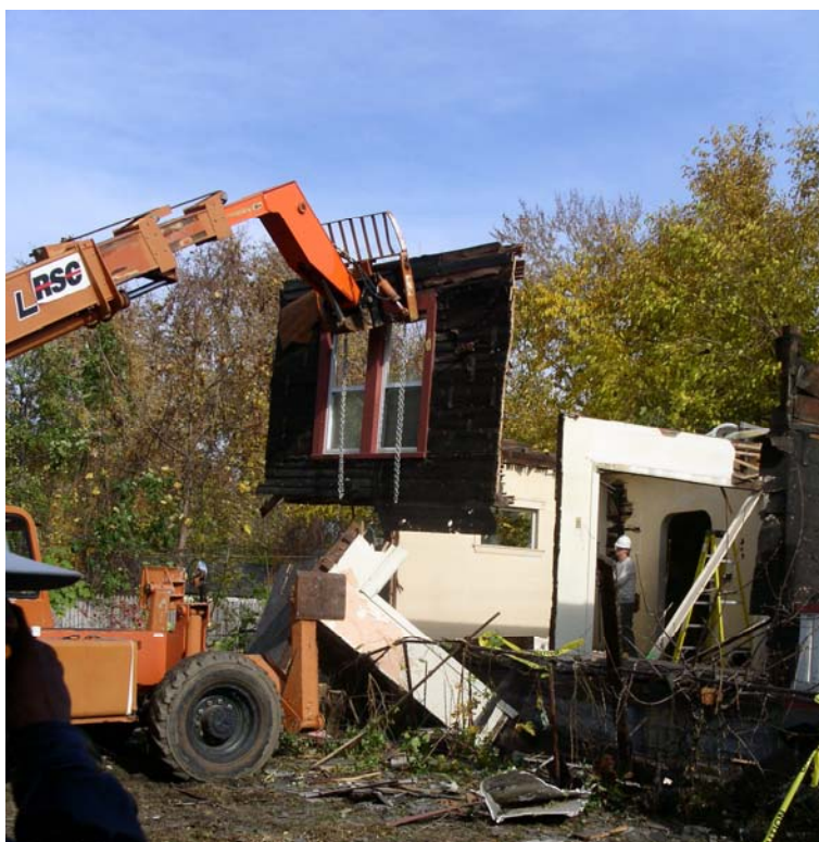
Photo 2 – Cleveland Deconstruction Initiative – Removal of House Panel
