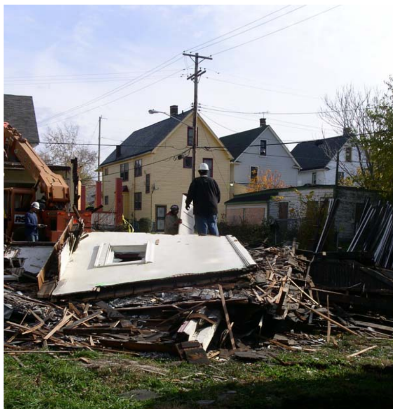
Photo 3 – Cleveland Deconstruction Initiative – Panel Placement for Hand Dismantling
