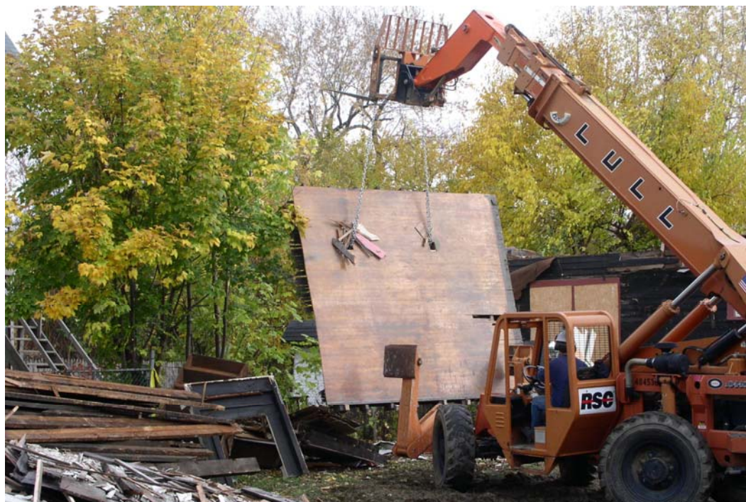
Photo 4 – Cleveland Deconstruction Initiative – Floor Removal
