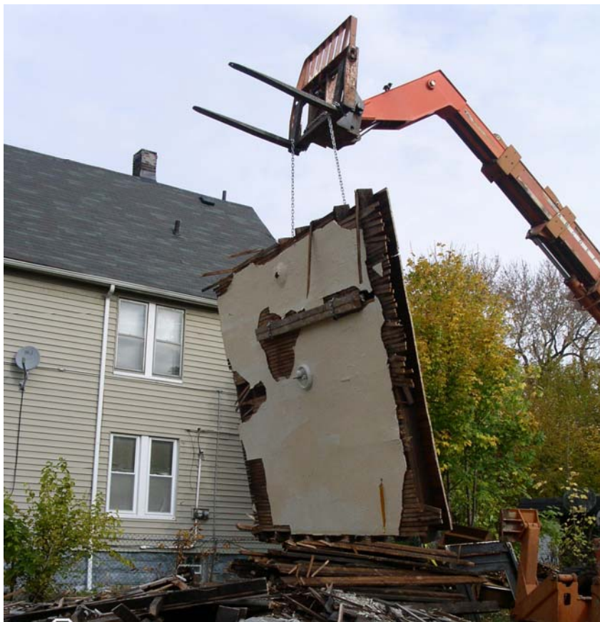
Photo 5 – Cleveland Deconstruction Initiative – Wall Removal
