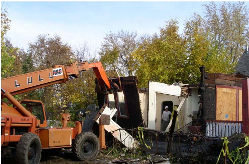
Photo 1 – Cleveland Deconstruction Initiative – Removal of House Panel
