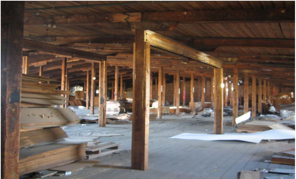
Photograph No. 1: Thornhill 7A (upstairs)—view of 6”x 6” timber column structure
