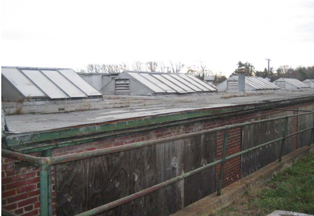
Photograph No. 5: Skylights on top of Allen-Morrison facility
