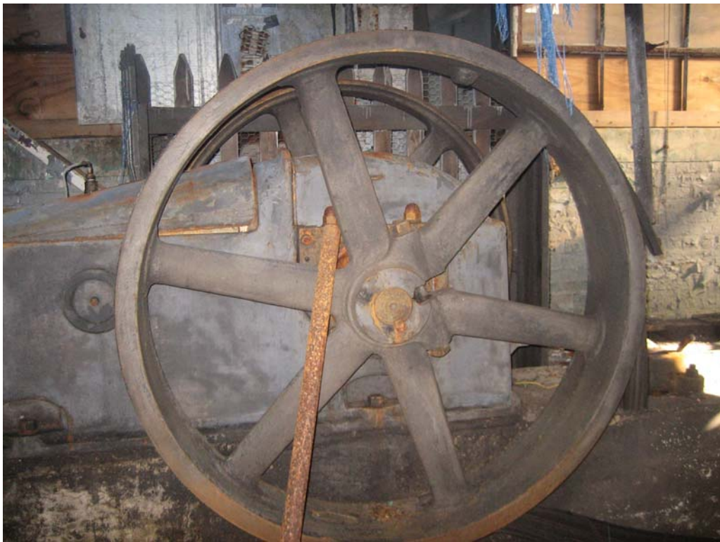
Photograph No. 12: Wheeled equipment in Allen-Morrison 1A
