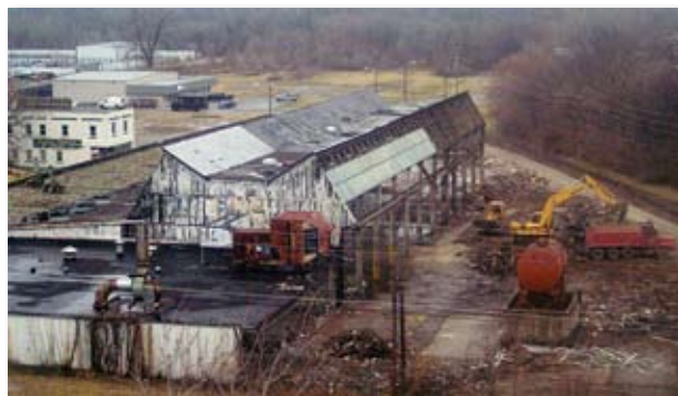
Prime Battery site before demolition
