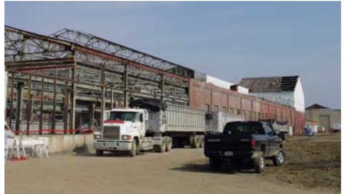
Construction activities at the former PPG Factory
