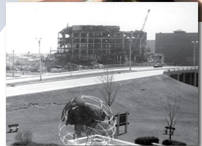
Demolition of the Former Chrysler Plant
