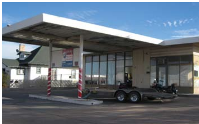
Gas station along Rt. 66 corridor
