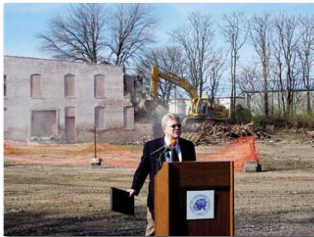
Demolition of the F.C. Cline Building
