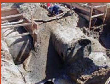
Underground Storage Tank removal
