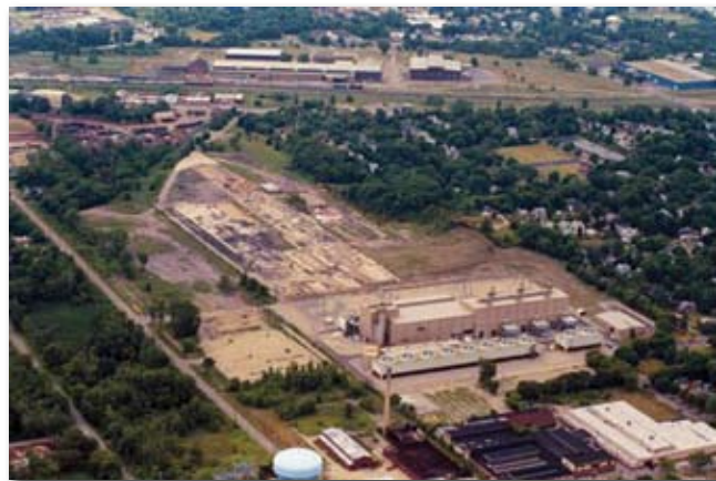
Aerial view of the redeveloped Goodyear property
