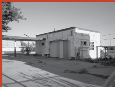
Gas station along Rt. 66 corridor
