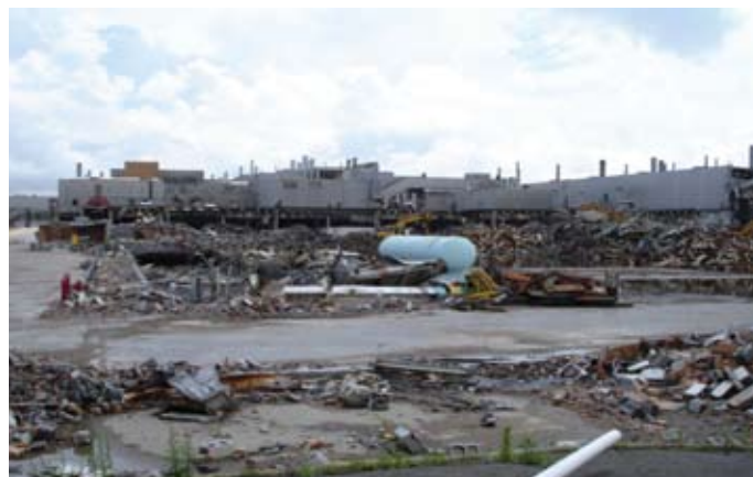
Demolition of the former GM Baltimore Plant
