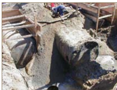
Workers unearth large underground storage tanks
