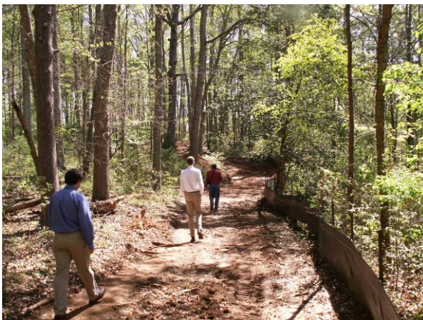
Trail Under Construction
