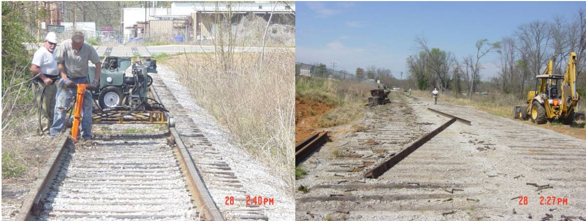
Rails Being Removed on former Greenville and Northern Line
