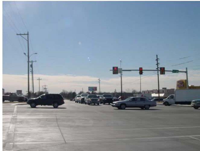
71st & Garnett Intersection; Garnett 61st to 71st
