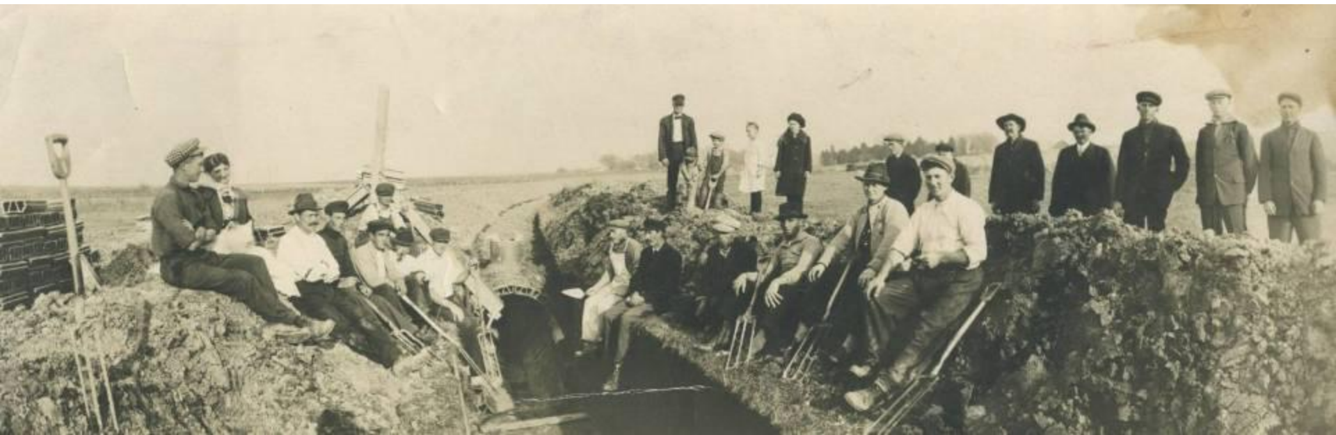
J.B. Crim Farm Nov 15 ,1916 end of 54 inch block tile in northern Boone Co.
