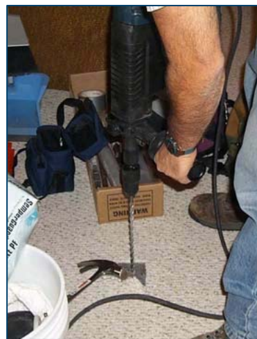
Figure 1: Drilling through slab
