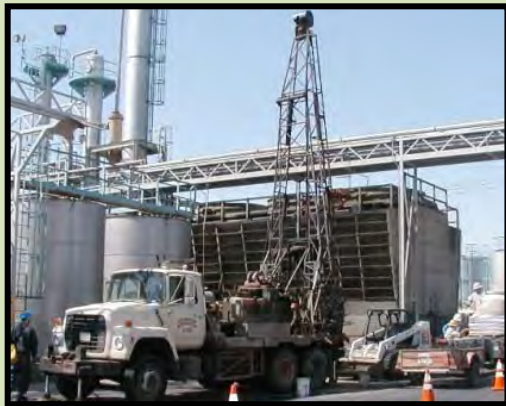
installation of 270 injection wells
