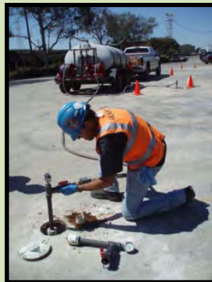
injections of nutrients in each well, 4 times per year
