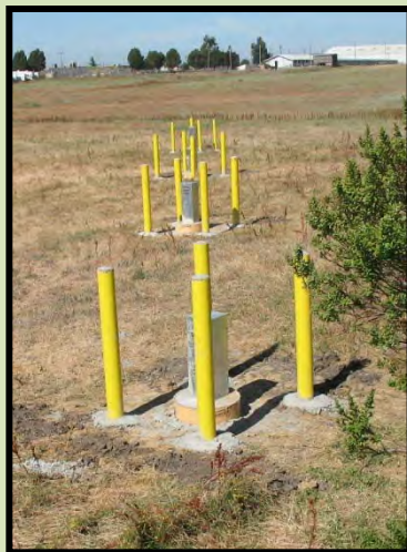
Biobarrier uses a row of 13 wells
