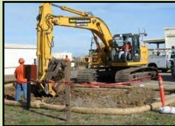
Contaminated soil removed and disposed as part of bioreactor construction
