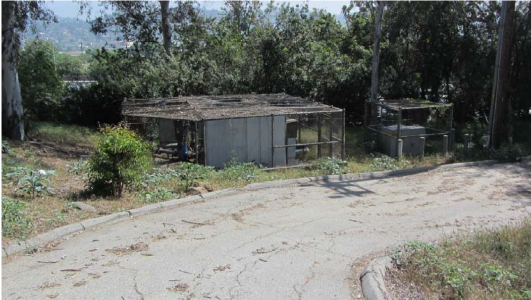
Figure 22. Existing Pump Station, View Northeast.
