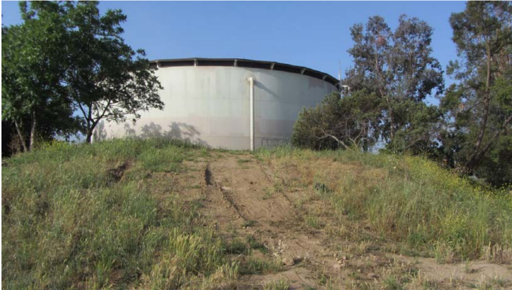
Figure 26. Existing 0.5 MG Steel Water Tank, View Southwest.
