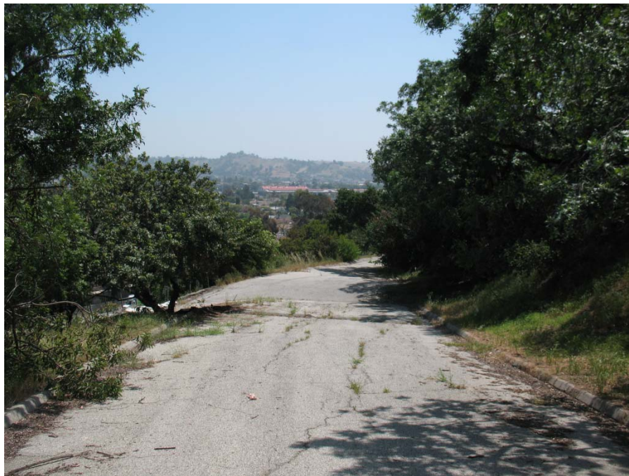
Photo 2. Photo of proposed recycled water pipeline route between Stadium Way and the proposed location for a new recycled water pumping station. Photo facing east.
