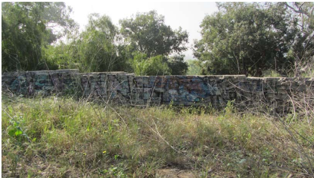
Figure 23. North Façade of Concrete Wall, View Southeast.
