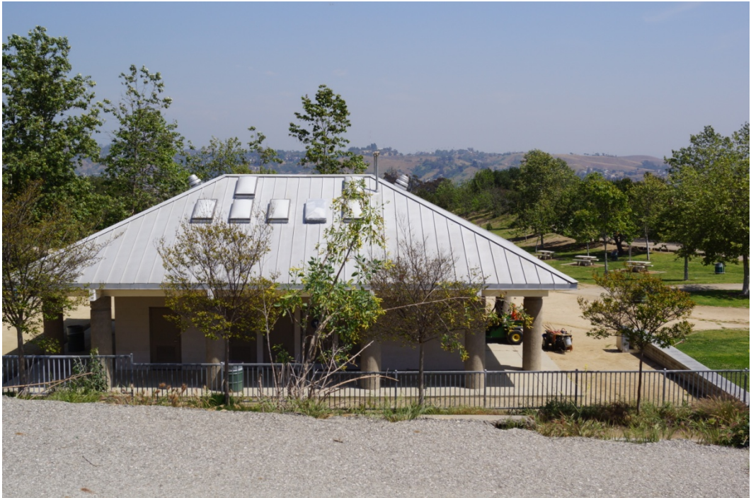
Figure 32. Public Restroom Facilities, View East
