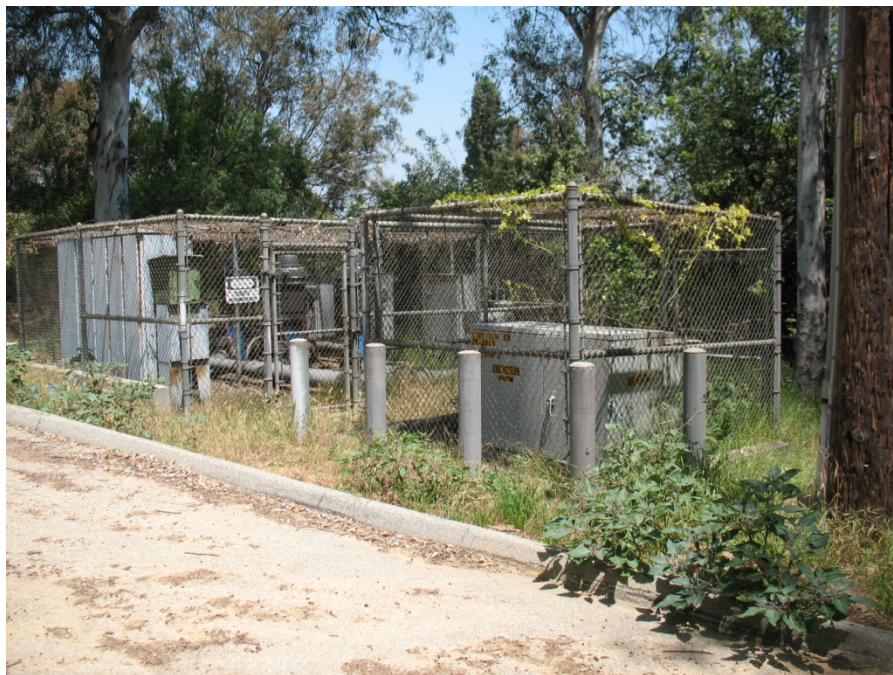
Photo 8. Existing electrical boxes and utilities are located immediately northwest of the proposed recycled water pumping station location. Photo facing north.
