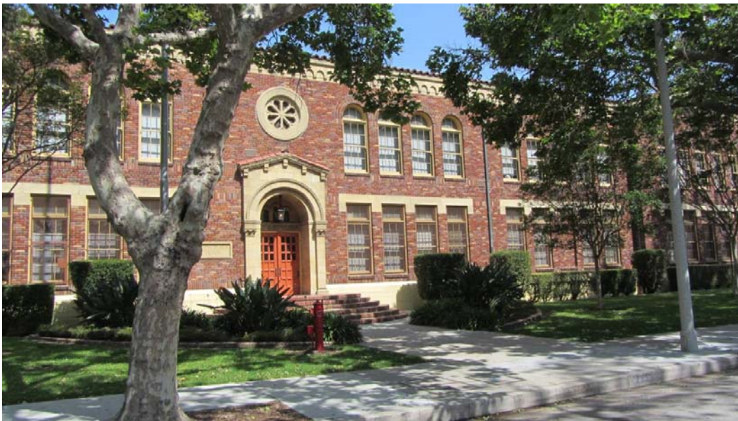
Figure 20. Dorris Place Elementary School, View Towards Northwest.
