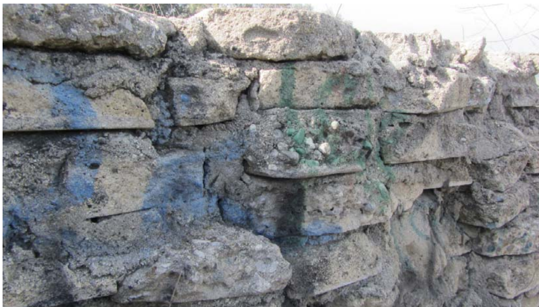
Figure 24. Close-up of Concrete Wall North Façade.
