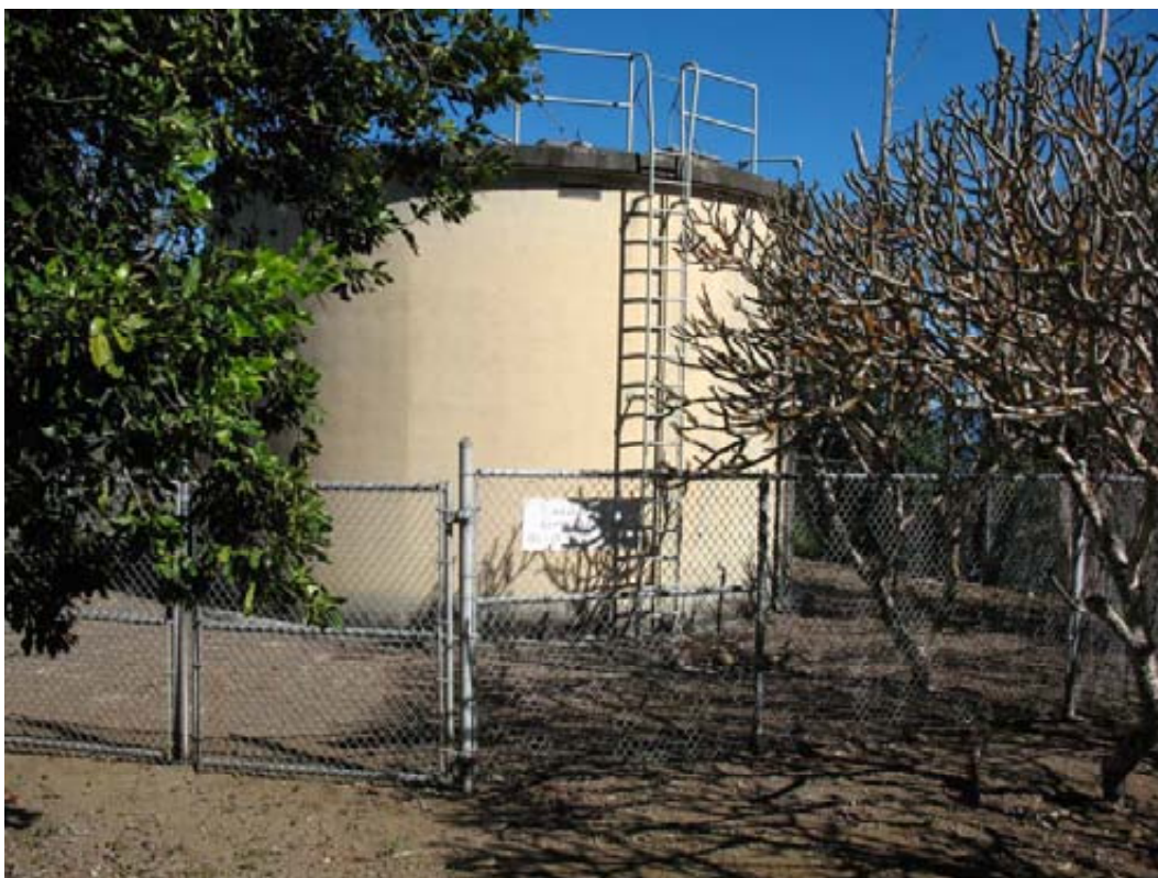
Figure 5. View to north of the existing 50,000 gallon water tank on TMK: 3-4-7-02:029.
