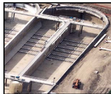
Figure 2.3: Oxidation Ditch
