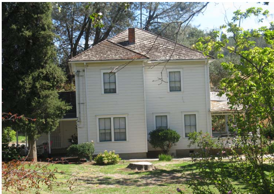
Photograph 2: Residence 1, camera facing northeast
