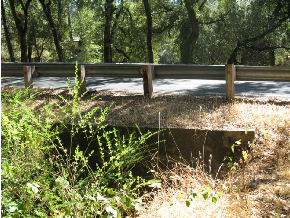
Photograph 4: Applegate Road and Boardman Canal Segment, camera facing south
