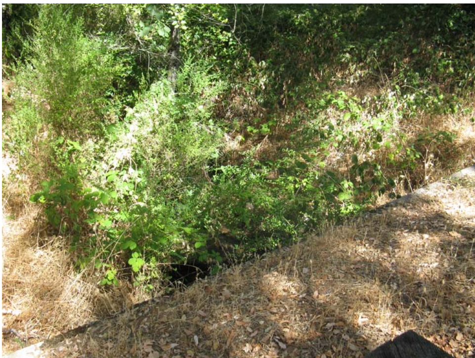
Photograph 5: Boardman Canal Segment from Applegate Road, camera facing northwest
