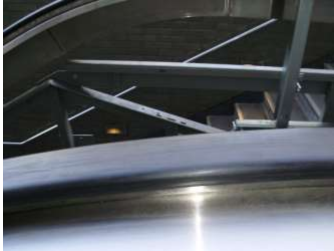
Figure 6-2. Close up of rubber handrail
