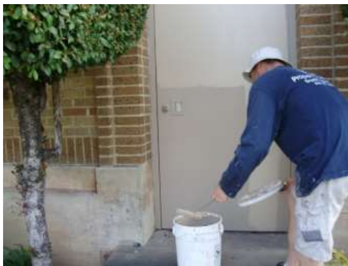
Figure 2-1. Contractor painting over metal door
