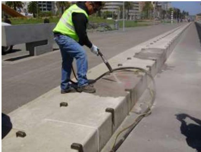
Figure 3-10. Glass blasting system removing spray paint from divider
