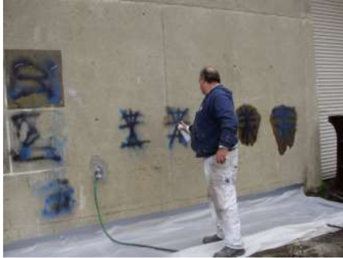
Figure 4-4. Port staff applying graffiti remover to concrete wall
