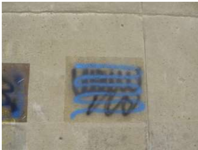
Figure 5-12. Coval coating on concrete wall with graffiti
