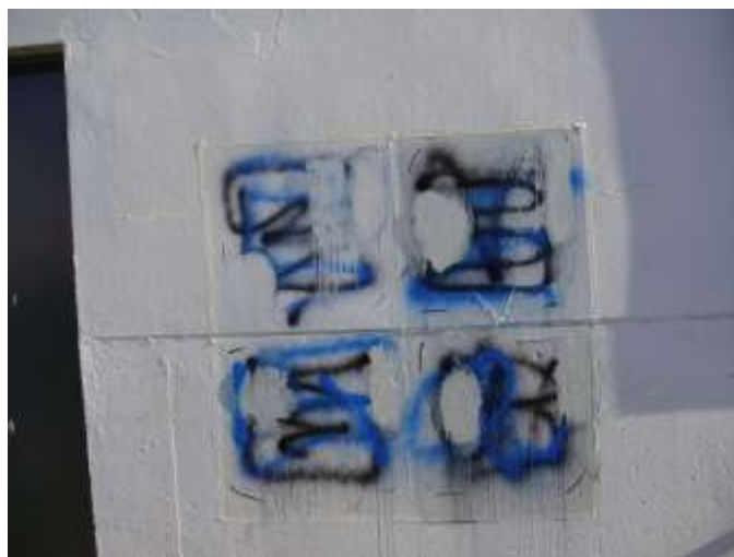
Figure 5-10. Graffiti resistant coatings on concrete after graffiti removal
