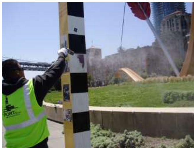
Figure 3-15. Glass blasting system removing sticker from pole
