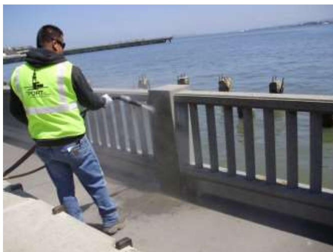
Figure 3-12. Glass blasting system removing spray paint from railing
