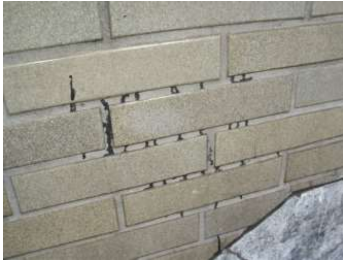
Figure 6-4. Graffiti on grout in underground train structure
