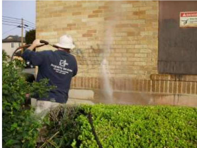
Figure 2-4. Contractor using soda blasting system
