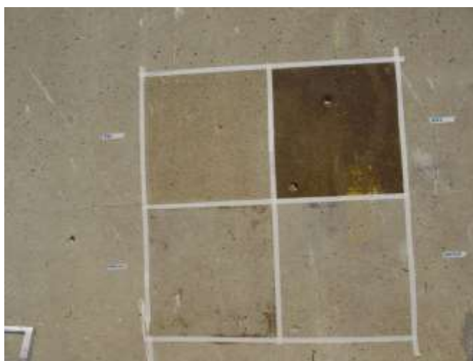
Figure 5-4. Graffiti resistant coatings on concrete wall
