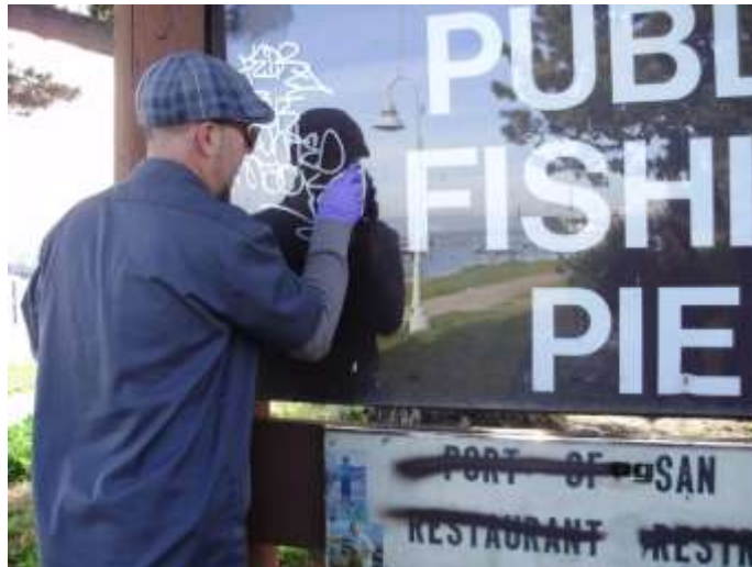
Figure 2-7. Port staff using graffiti remover on plexiglass
