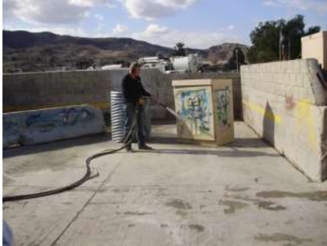
Figure 3-21. Glass blasting system removing graffiti from metal box
