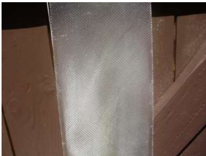
Figure 5-17. Lighting fixture with pebbled surface
