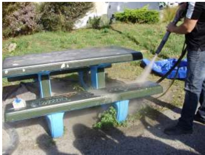
Figure 3-4. Blasting system removing graffiti from picnic table
