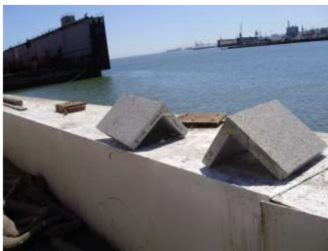
Figure 5-6. Graffiti resistant coatings on granite pieces
