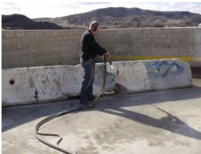
Figure 3-18. Dry ice blasting system removing paint from concrete barrier
