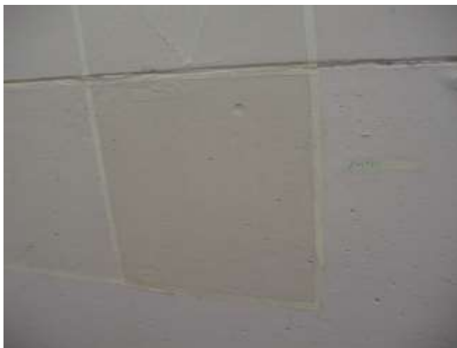
Figure 5-5. Graffiti resistant coatings on painted stucco
