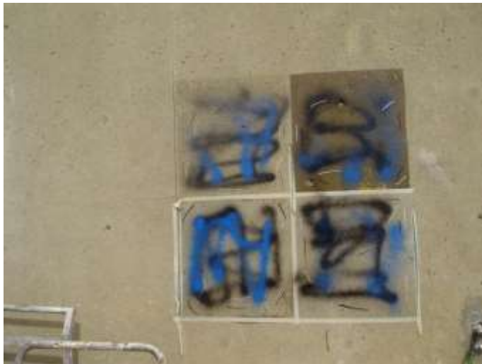
Figure 5-7. Graffiti resistant coatings on concrete with graffiti
