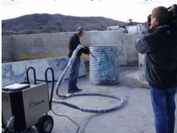
Figure 3-19. Dry ice blasting system removing graffiti from metal component
