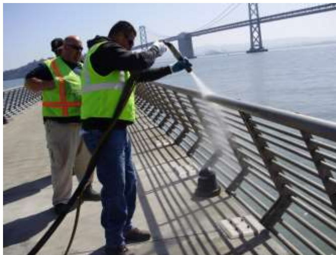
Figure 3-7. Dry ice blasting system removing graffiti from railings
