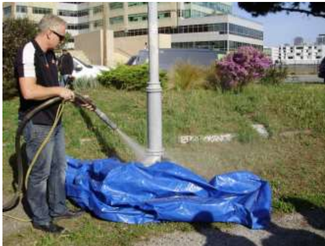
Figure 3-3. Blasting system removing graffiti from lamppost
