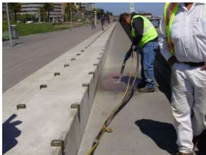
Figure 3-11. Glass blasting system removing spray paint from walkway
