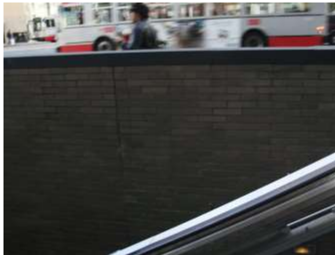
Figure 6-1. Rubber handrail on escalator
