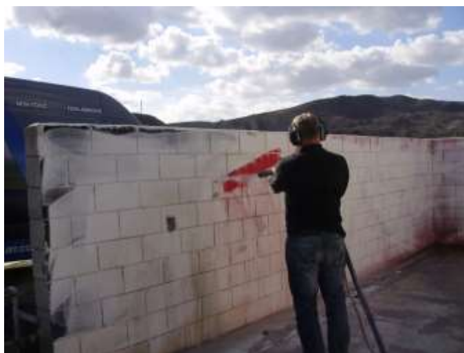
Figure 3-20. Glass blasting system removing paint from concrete wall
