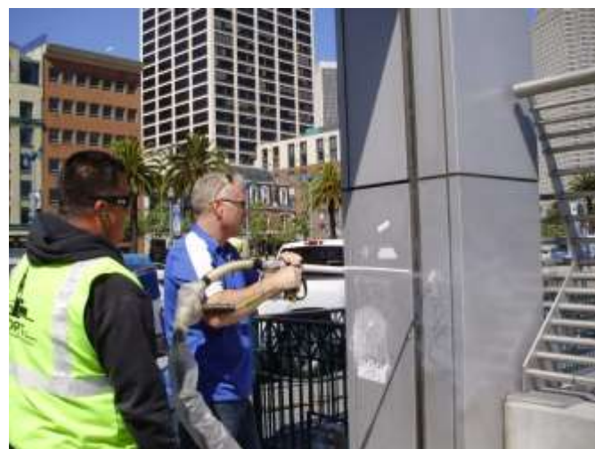
Figure 3-9. Dry ice blasting system removing spray paint from post
