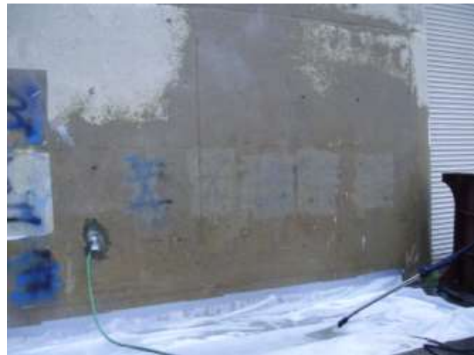
Figure 4-6. Concrete wall after rinsing
