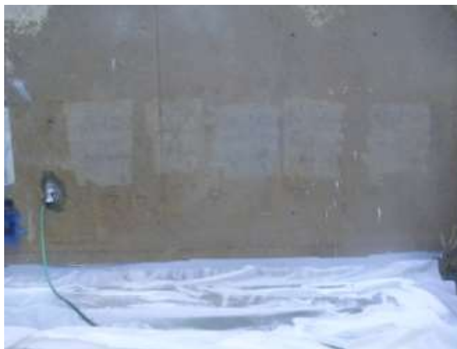
Figure 4-7. Concrete wall after graffiti removal
