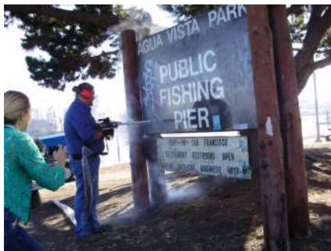
Figure 3-17. Dry ice blasting system removing graffiti from billboard
