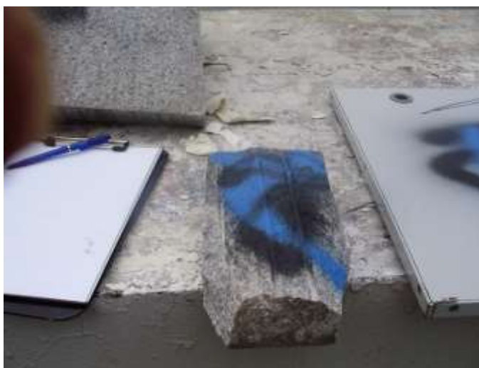
Figure 5-13. Coval coating on granite with graffiti
