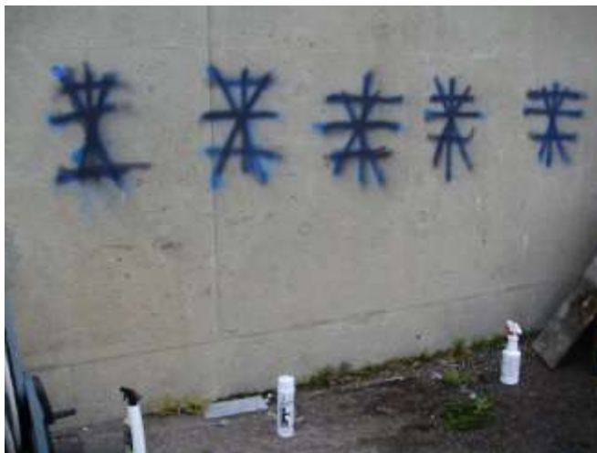
Figure 4-3. Port concrete wall with spray paint applied
