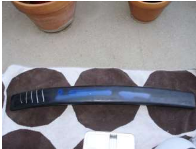
Figure 6-3. Rubber handrail with graffiti
