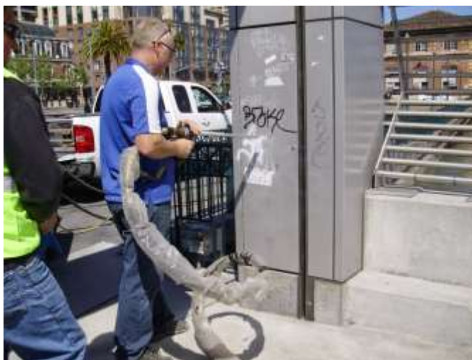
Figure 3-8. Dry ice blasting system removing graffiti from post
