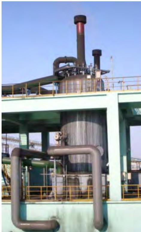
Picture of process water degasser
