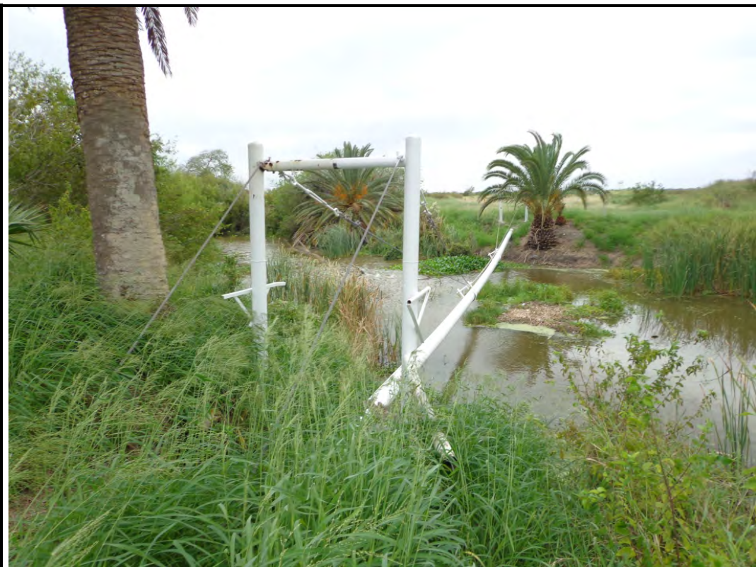
Photograph: 25 W view of pipeline crossing Green Lake Ditch habitat. voestalpine Texas, LLC ERM La Quinta Site San Patricio County, TX
