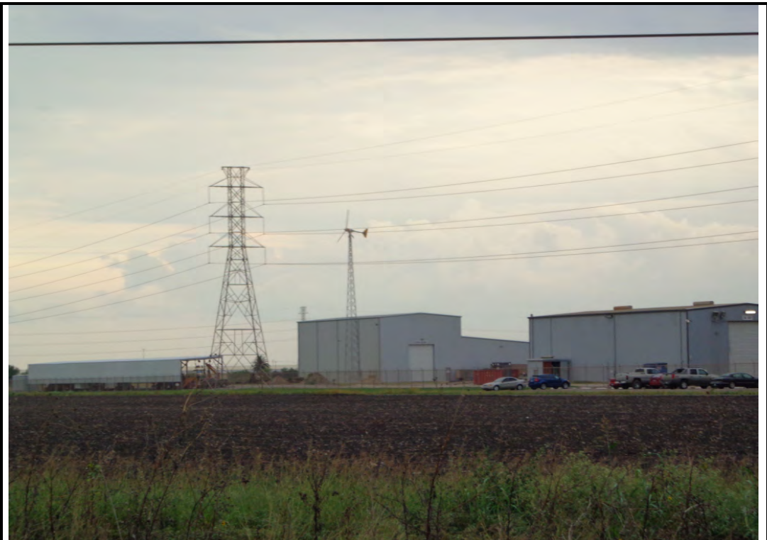
Photograph: 51 View W from La Quinta Road to light industrial and commercial buildings, power transmission lines, and wind turbine located north of the Project site and immediately south of TX-35.
