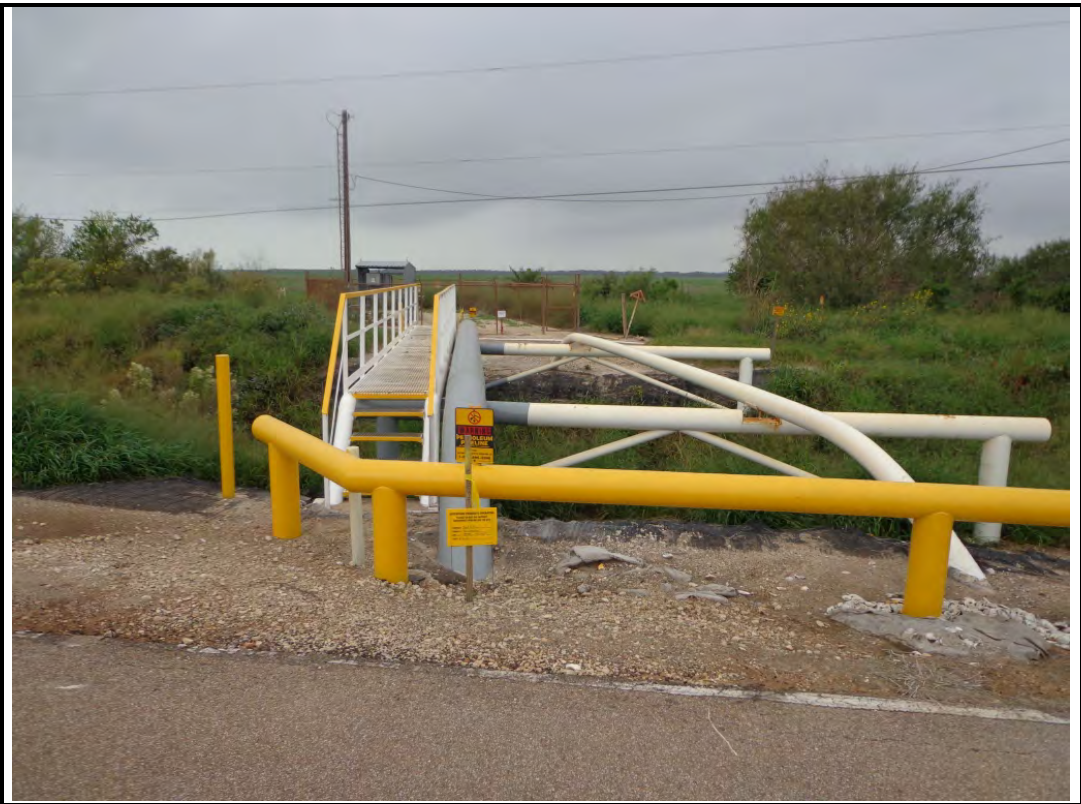
Photograph: 5 | W view from La Quinta Road of Air Liquide and Enterprise Products pipelines crossing La Quinta Ditch.
