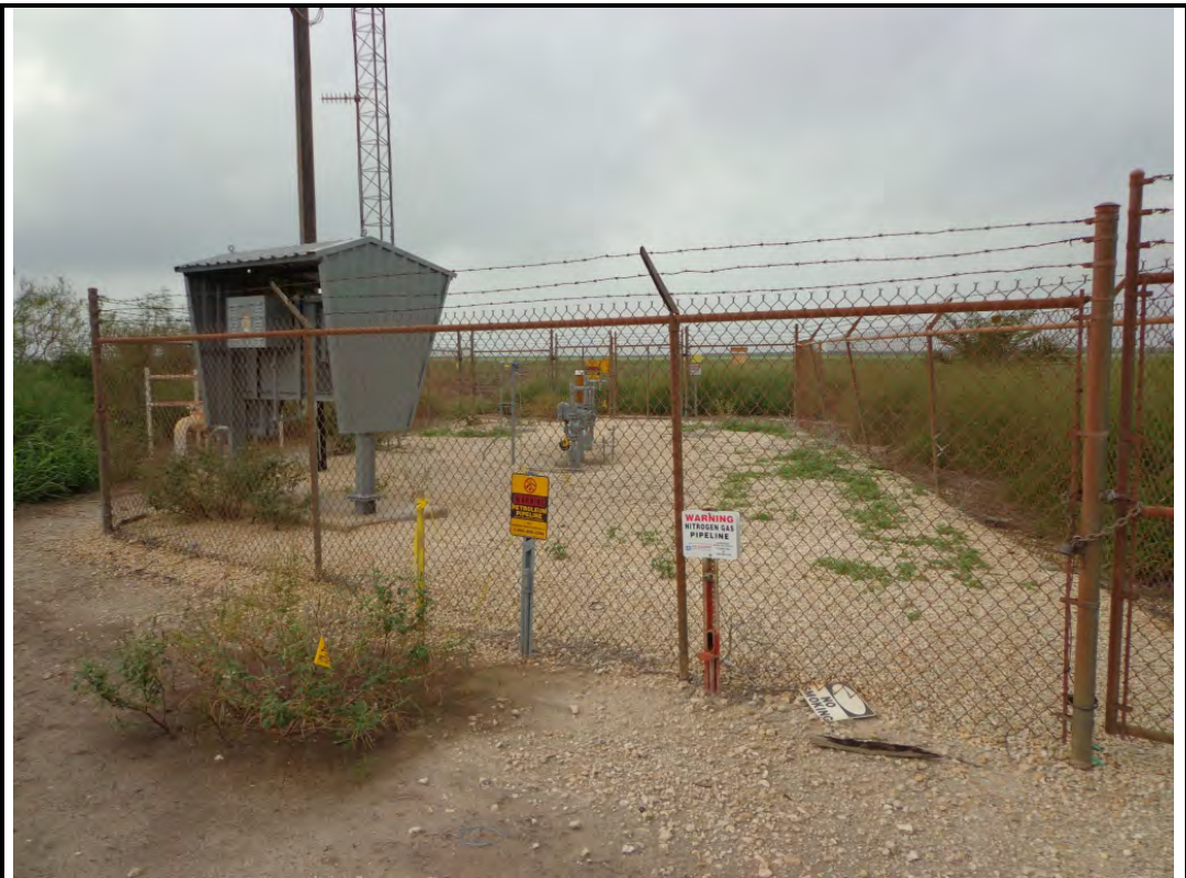
Photograph: 6 | SW view of Air Liquide, Enterprise, and Southcross pipelines and remote monitoring station at eastern boundary of Project site.
