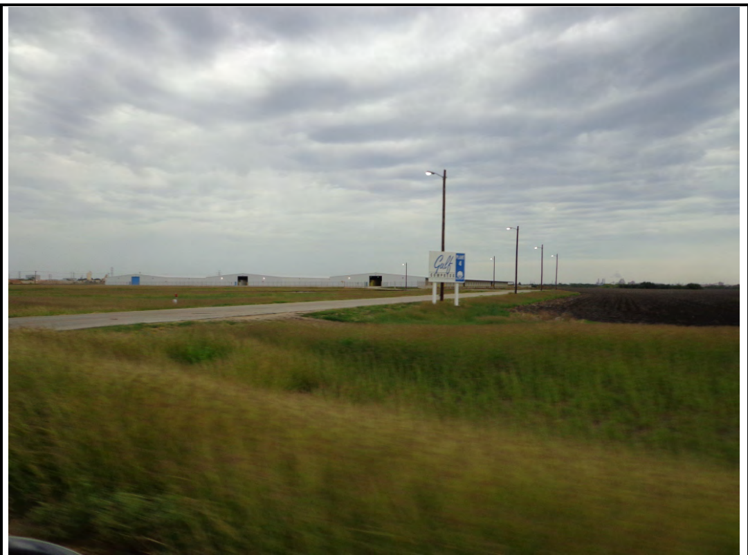
Photograph: 48 E view of the Gulf Compress cotton storage facility from US Hwy 181 frontage road. voestalpine Texas, LLC ERM La Quinta Site San Patricio County, TX
