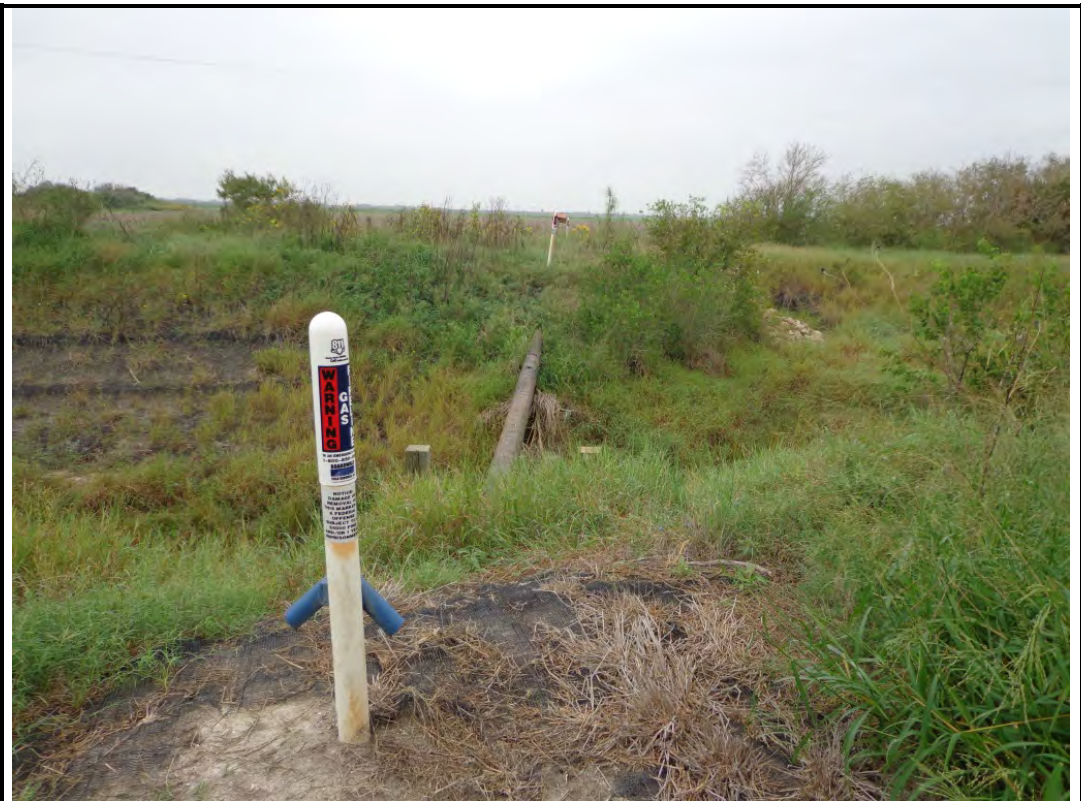
Photograph: 7 | NW View of Boardwalk Pipeline crossing La Quinta Ditch at southeast boundary of Project site.
