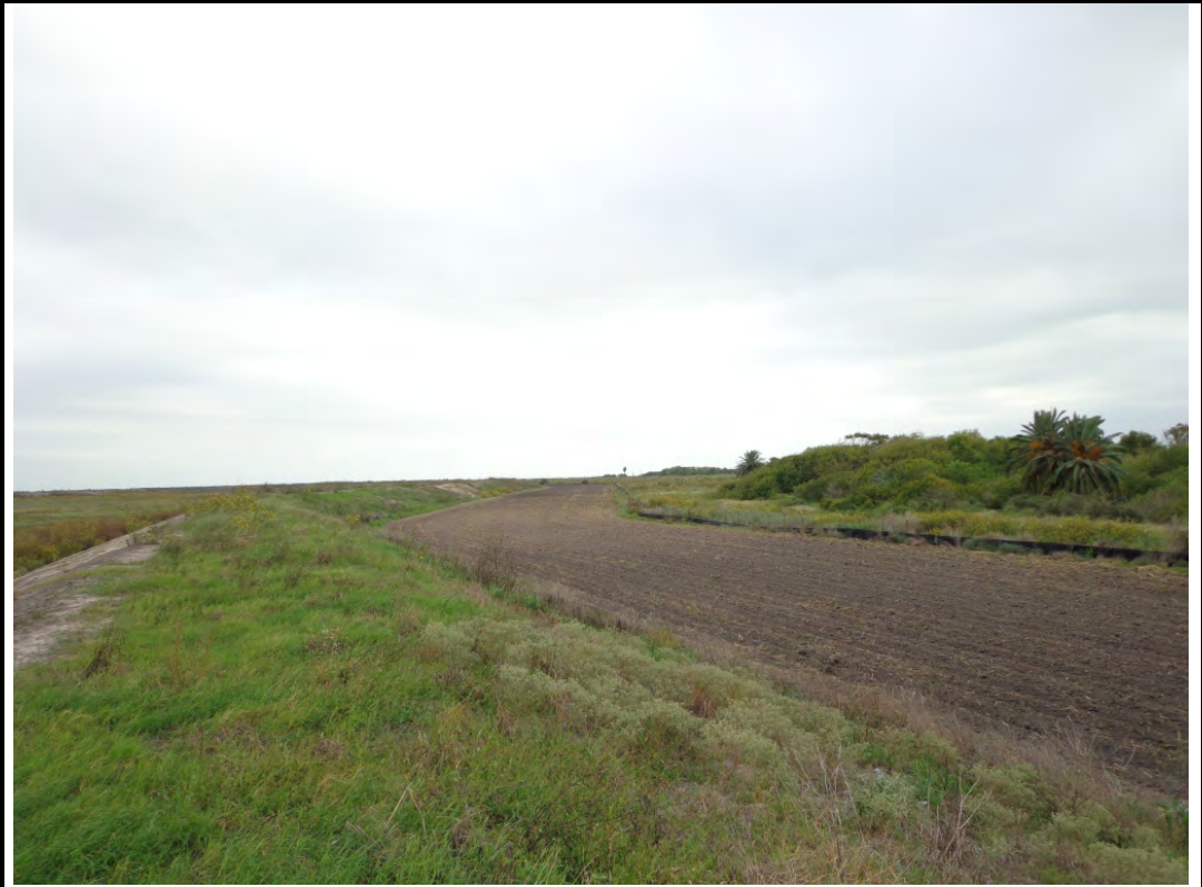
Photograph: 36 | S view of western berm of southernmost spoil pond.
