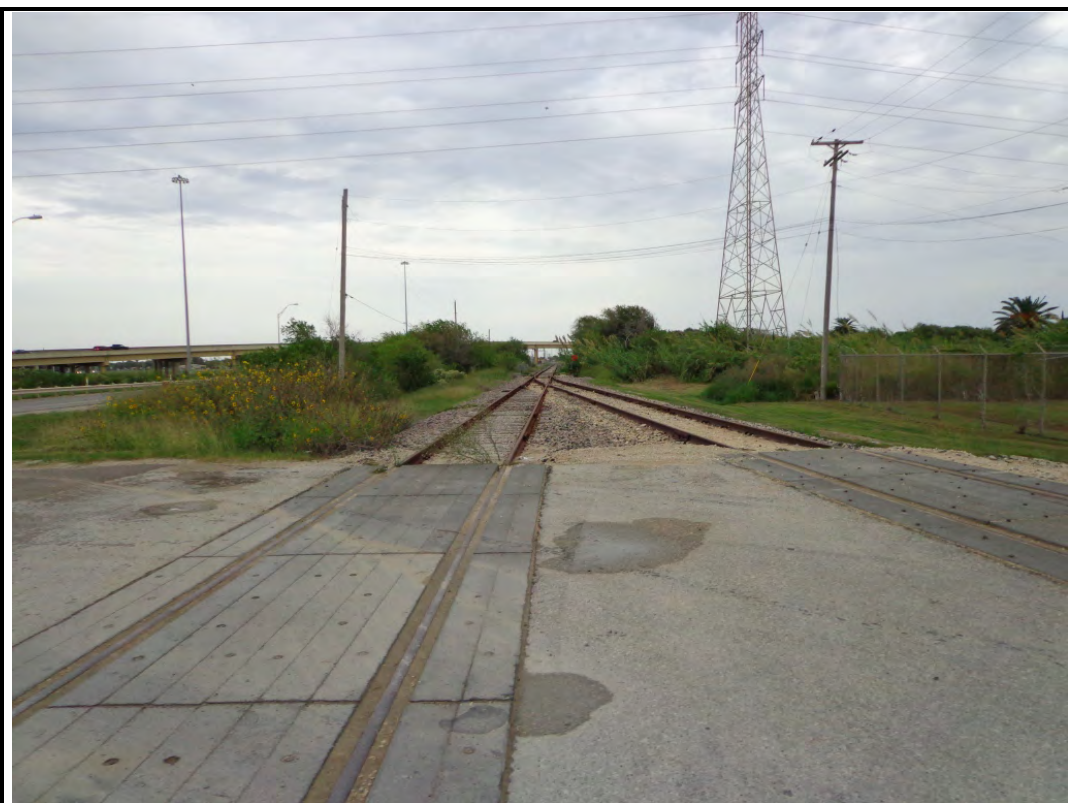
Photograph: 50 | View to N of rail west of site leading into Gregory, TX.
