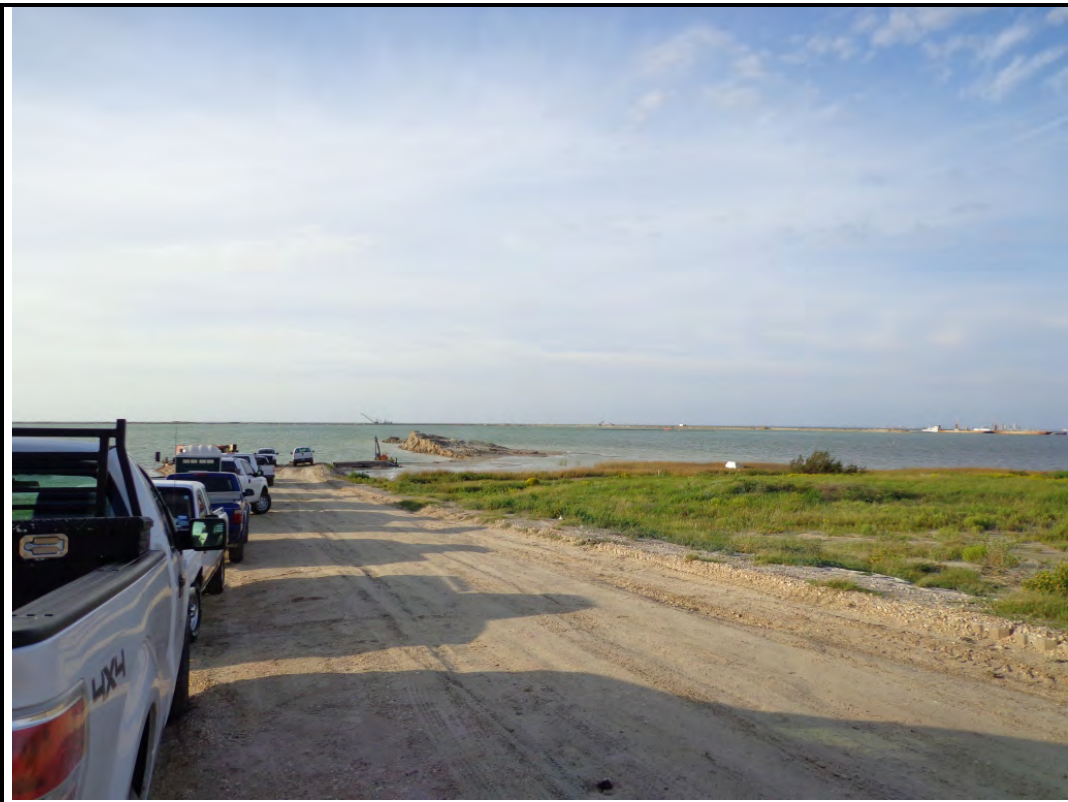
Photograph: 59 | S view of access road/landing area for dredging operations, POCCA terminal area, and Corpus Christi Bay.
