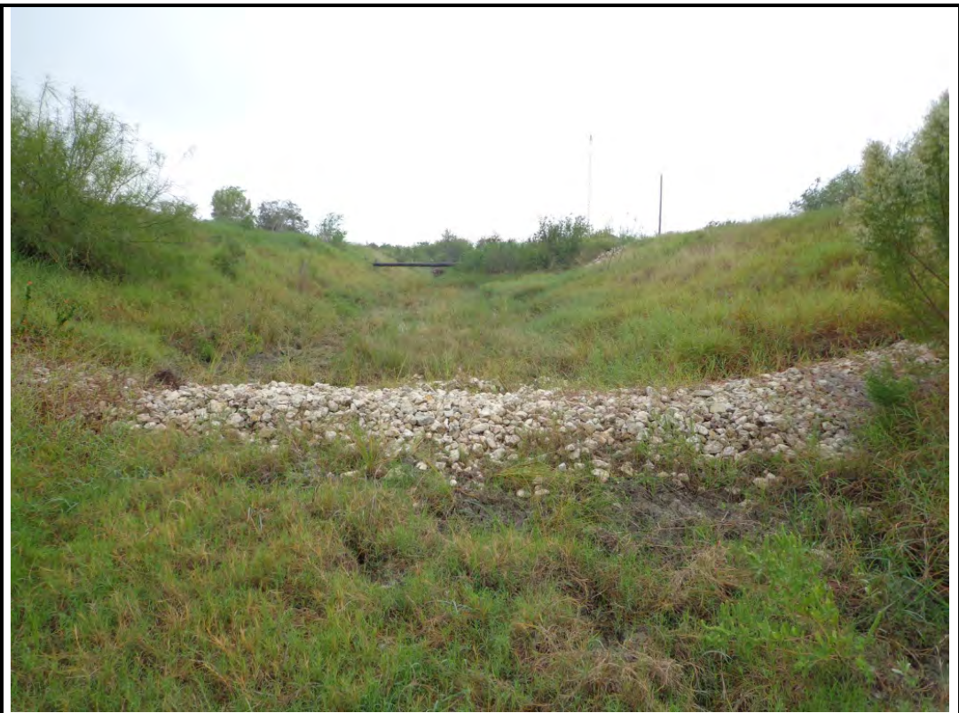
Photograph: 14 | S view of erosion control present in la Quinta Ditch.
