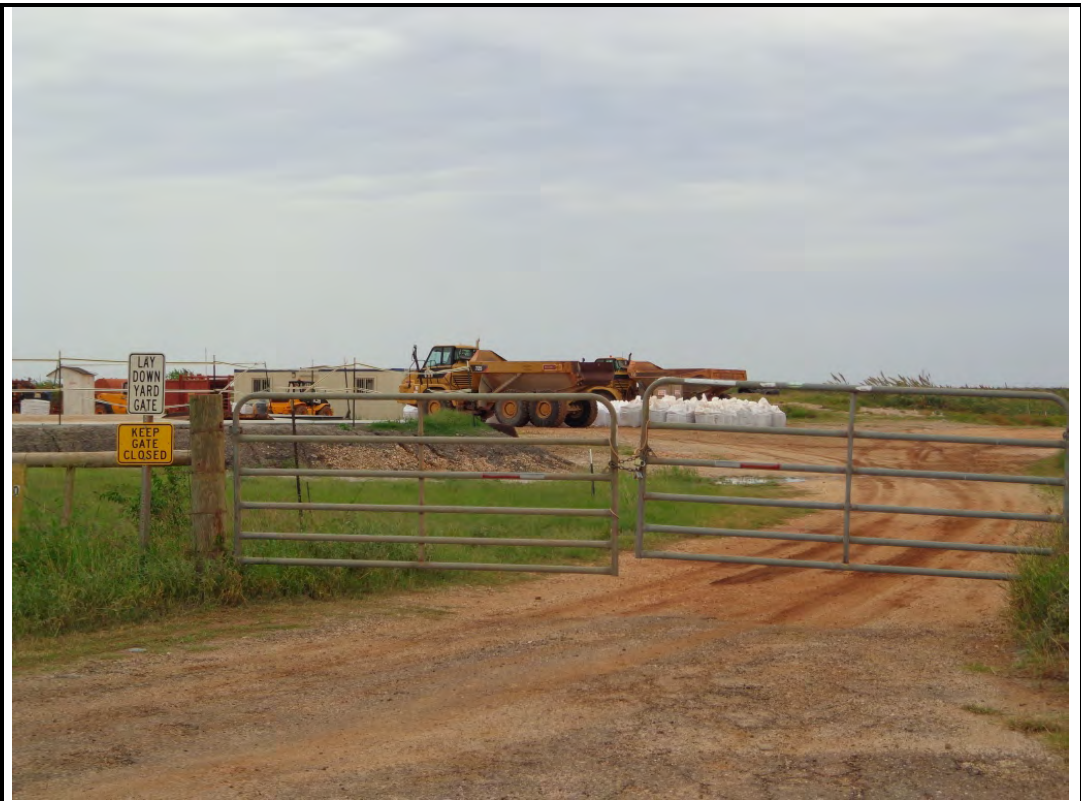
Photograph: 54 View E from La Quinta Road of gated entrance to a laydown yard on adjacent Sherwin Alumina property.
