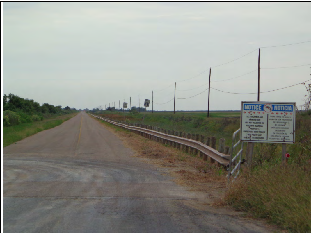
Photograph: 1 View SE of entrance to La Quinta Road and eastern boundary of Project site from TX-35.
