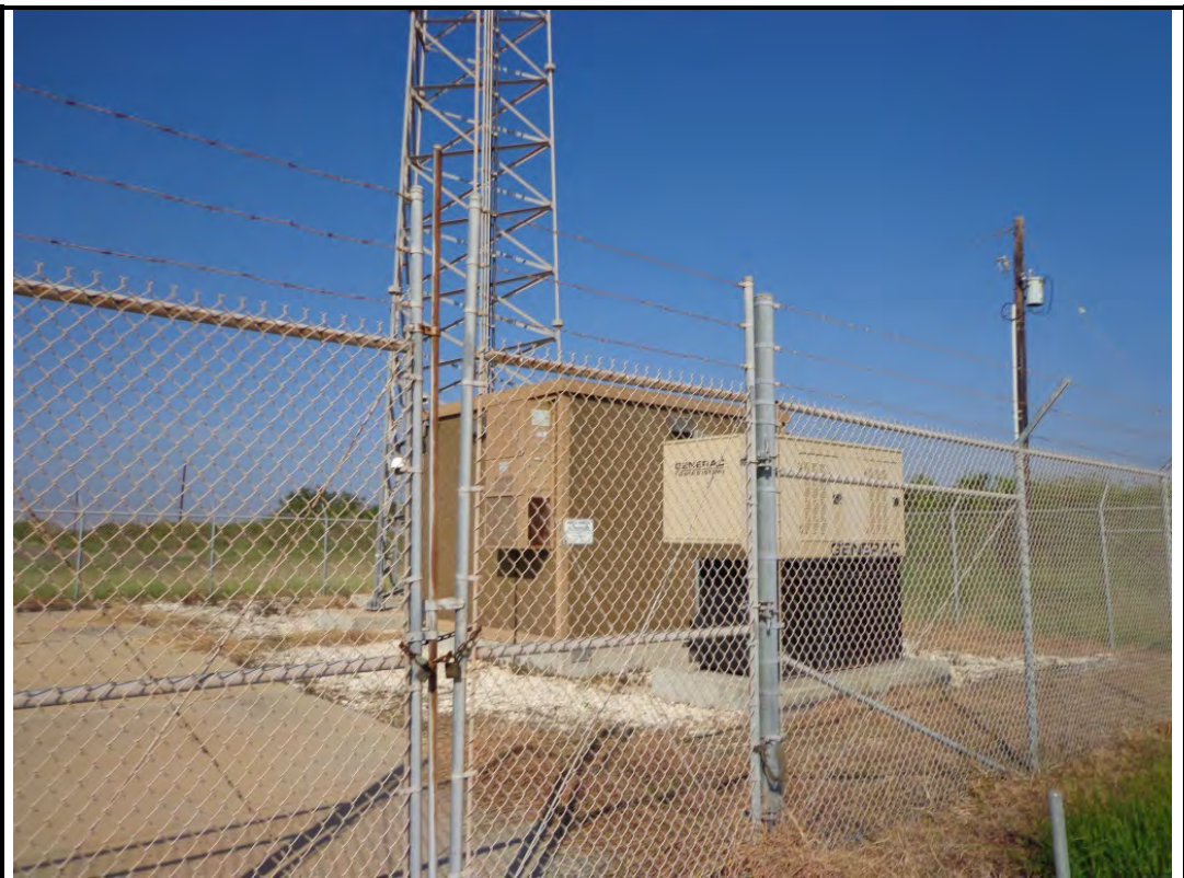
Photograph: 8 | View NE of communications tower located at southeastern portion of Project site.
