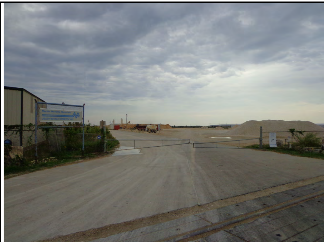
Photograph: 49 | SE view of Martin Marietta Materials from US Hwy 181 frontage.
