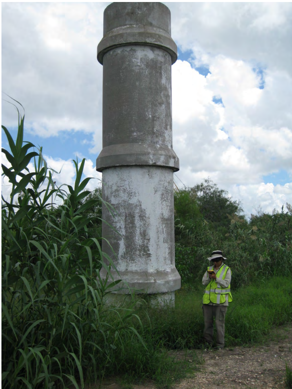
Figure 17. Concrete standpipe
