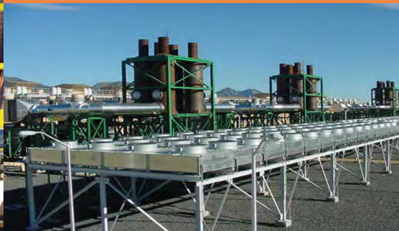
Closed-loop cooling system with radiators
