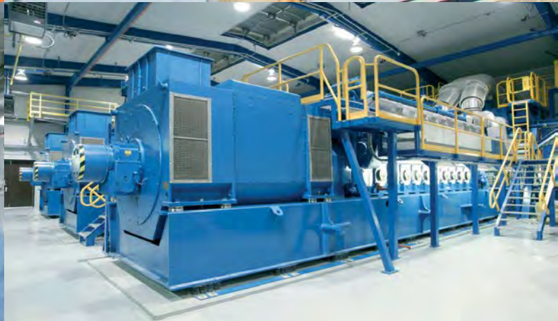
The generating set
