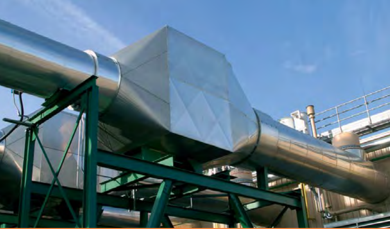
Selective Catalytic Reduction unit (SCR)
