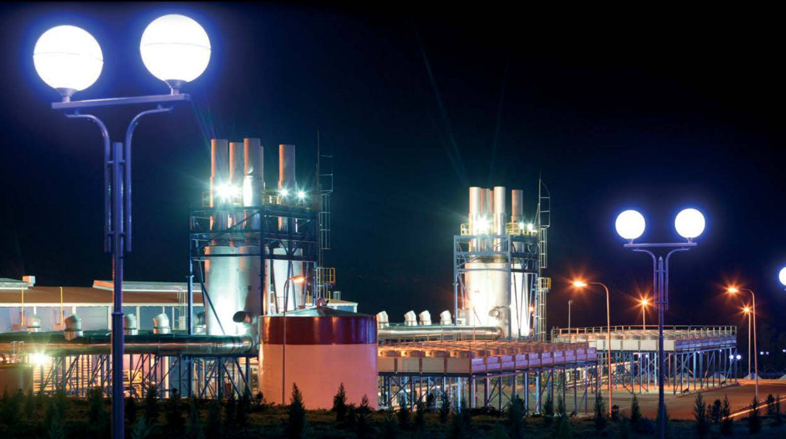
The Sheki power plant in Azerbaijan is equipped with 10 x Wärtsilä 20V34SG engines.
