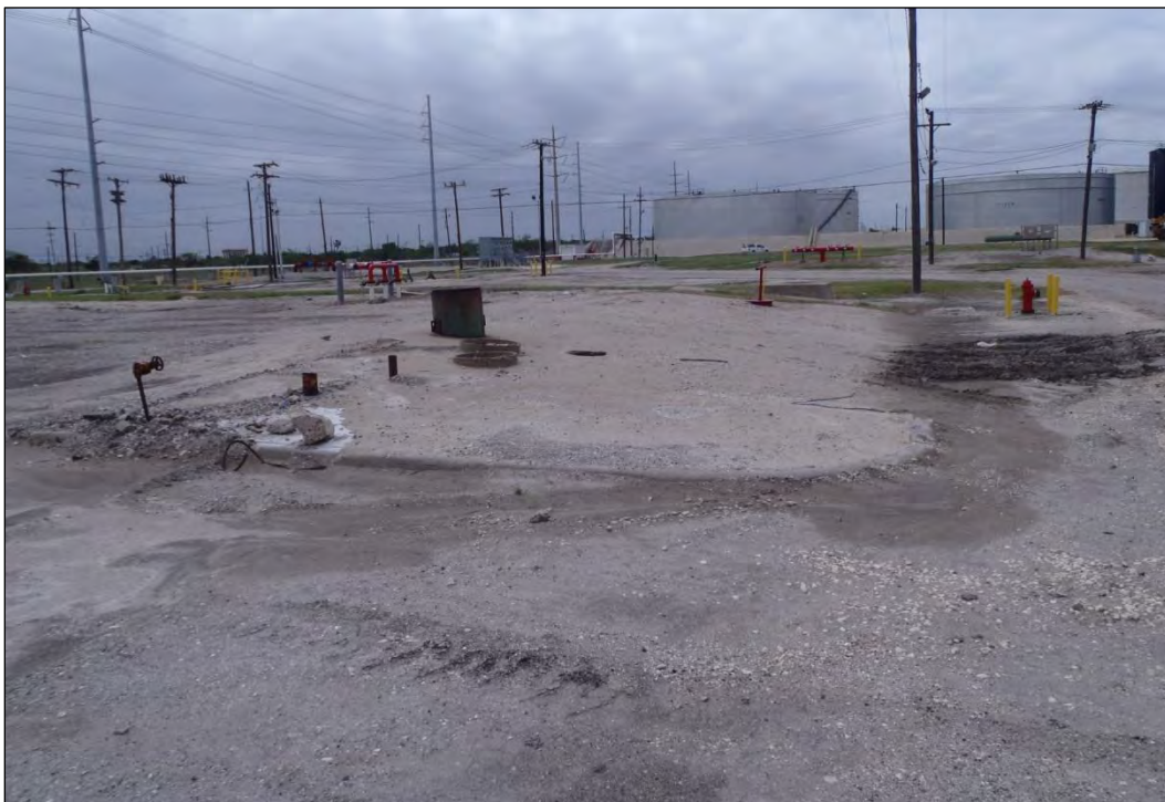
Figure 5. Typical View within Existing Corpus Christi Terminal
