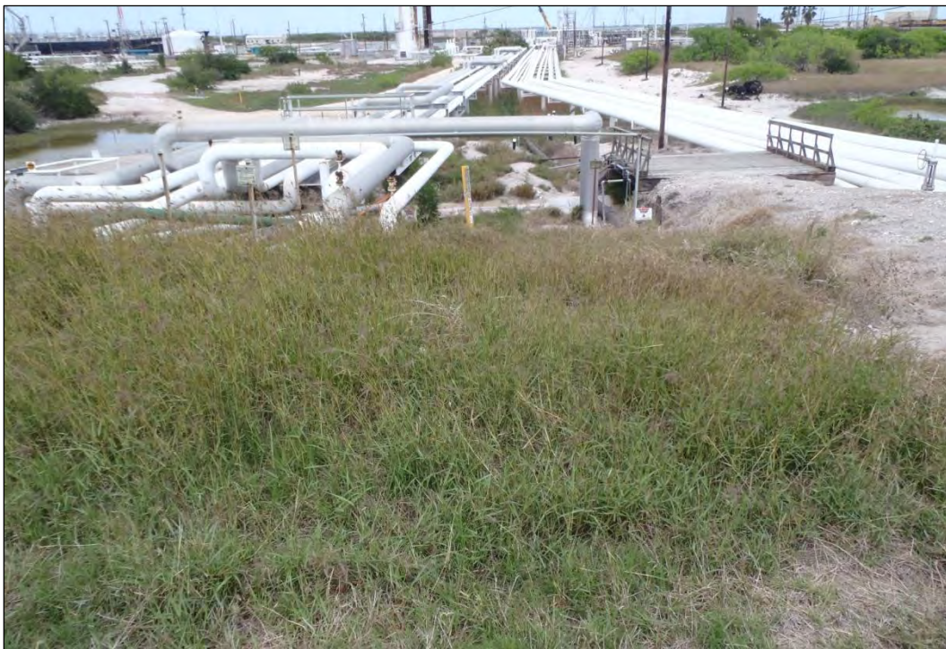
Figure 7. View of Existing Aboveground Pipe Racks near Dock
