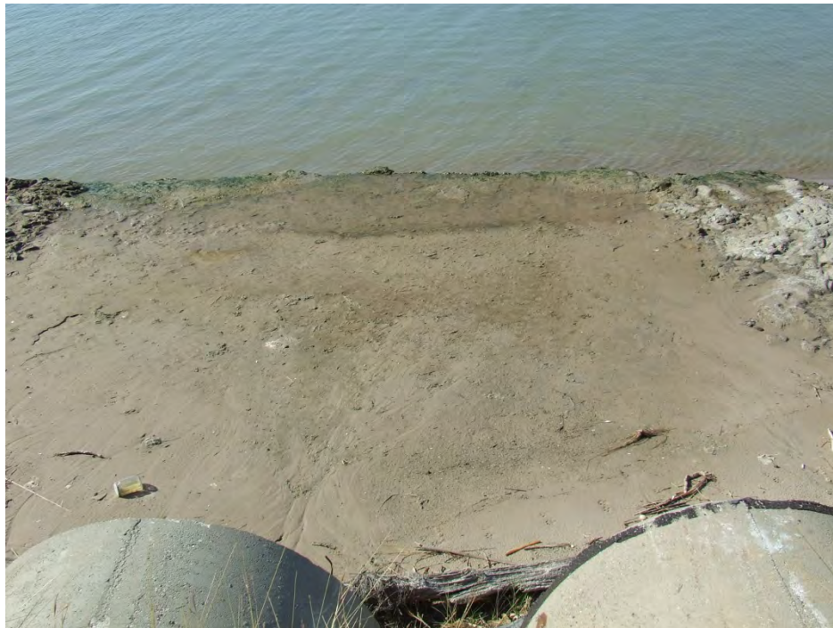
Photograph 8: November 6, Looking southwest at the outfall of the onsite trapezoidal flow-way into the Viola ship channel.
