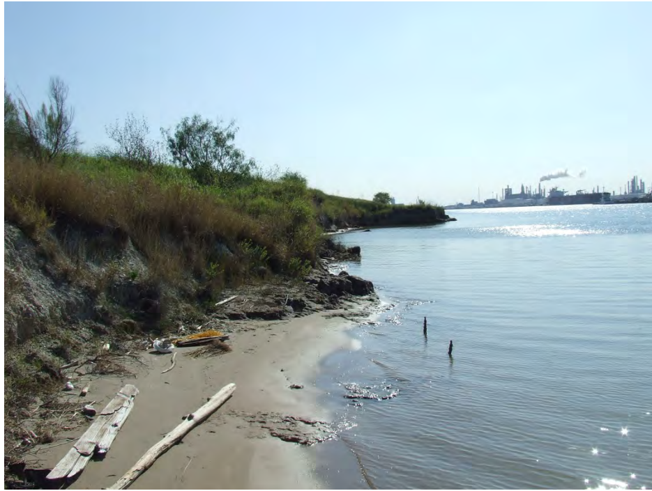
Photograph 9: November 6, Looking southeast at typical view of Viola ship channel shoreline.
