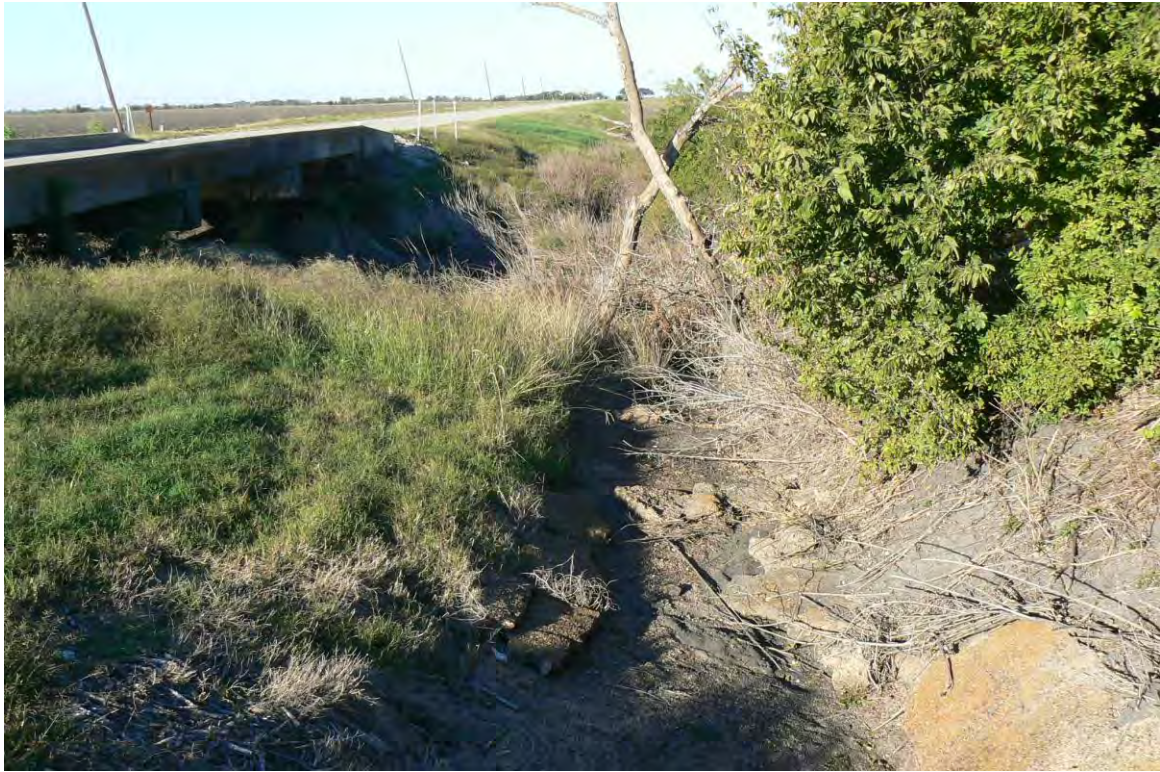
Photo 2. Dry swale draining west into Juanita Creek. Prairie rose in the upper right corner.
