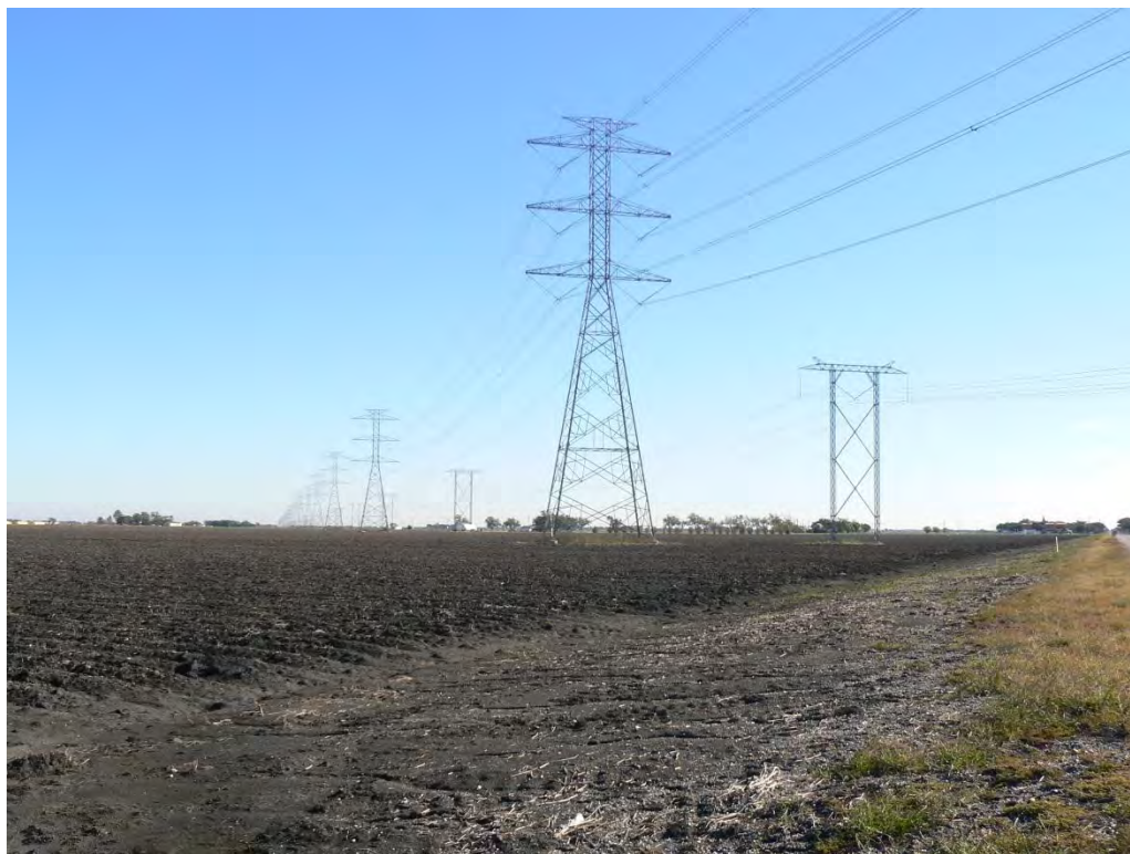
Photo 11. Southwest corner of the property looking northeast. The 345 kilovolt transmission line in the middle foreground and the distribution line in the right foreground.
