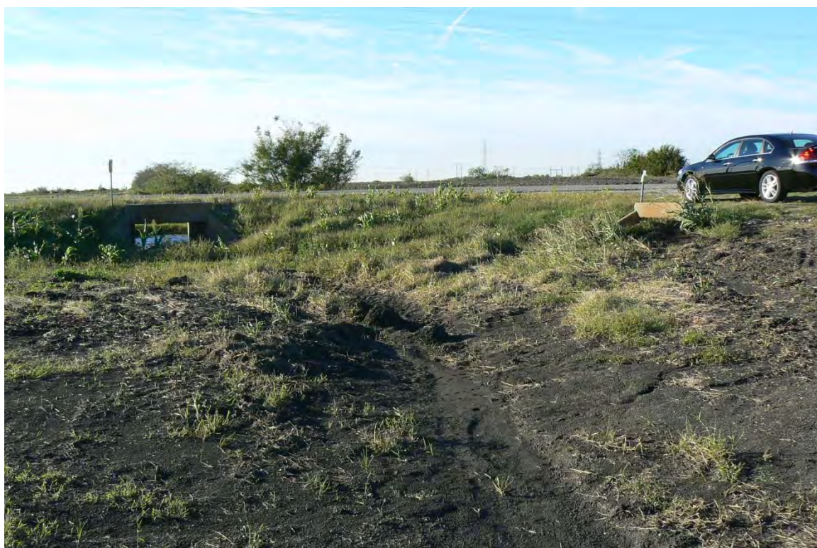
Photo 4. Culverts for swales just east of Juanita Creek looking south to Farm to Market Road 441.
