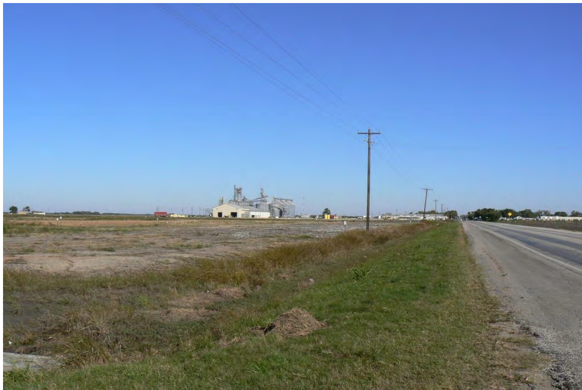
Photo 7. Northeast corner of the property looking north at the grain coop and State Route 71.
