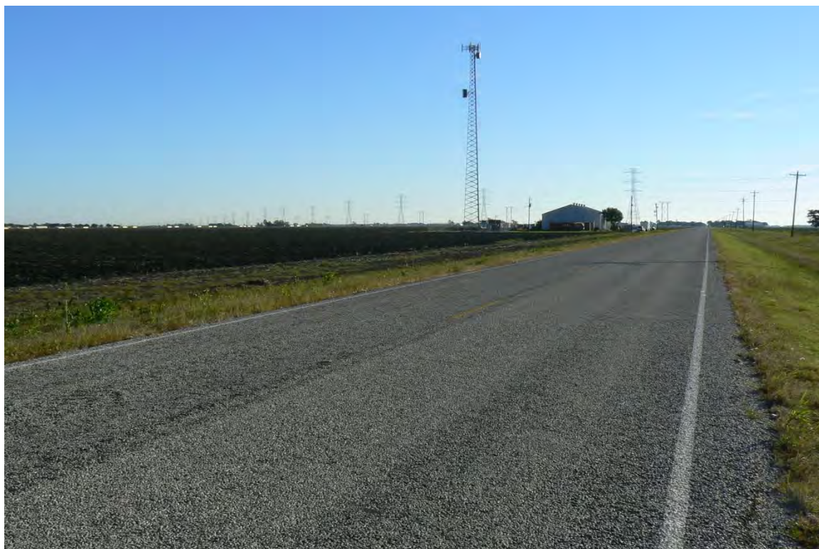
Photo 6. Offsite along Farm to Market Road 441 looking northeast at the cell tower.
