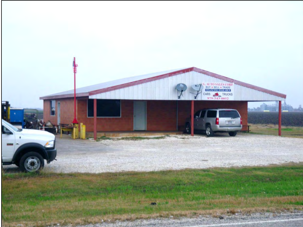
IMGP1683: Looking north at Archit-1 (14543 S. FM 441). (C. Borstel, Tetra Tech, December 4, 2013)
