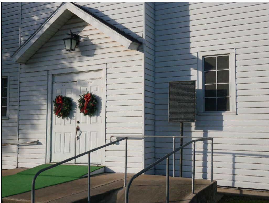
IMGP1371: Looking north-northwest at front (south) entrance to Danevang Lutheran Church. Marker recounting history of Lutheran Church in Danevang is to right of door. (C. Borstel, Tetra Tech, December 2, 2013)
