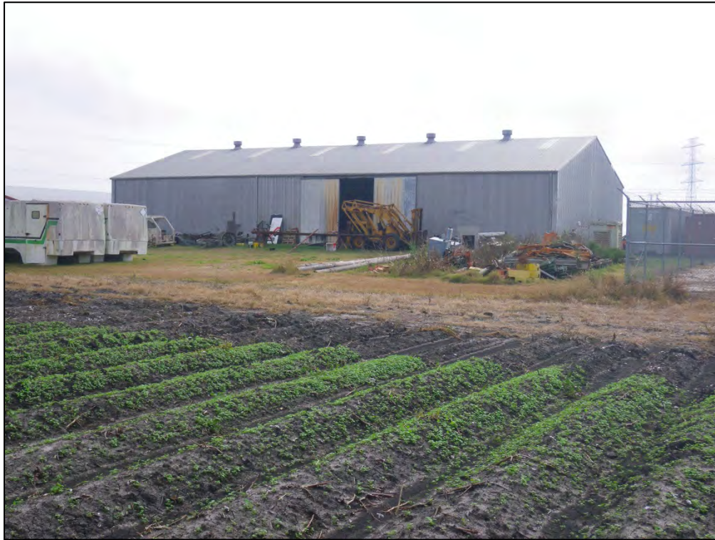
IMGP1608: Looking south-southeast at Archit-1 (14543 S. FM 441). (C. Borstel, Tetra Tech, December 4, 2013)
