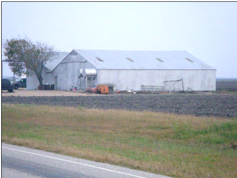
IMG1686: Looking southeast at Archit-2 ([no number] S. FM 441). Ca. 1960 section of metal-clad pole barn is at right (C. Borstel, Tetra Tech, December 4, 2013)
