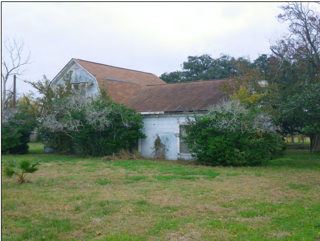
IMGP1728: Looking northeast at main house, Archit-3 (12177 SR 71). (C. Borstel, Tetra Tech, December 4, 2013)
