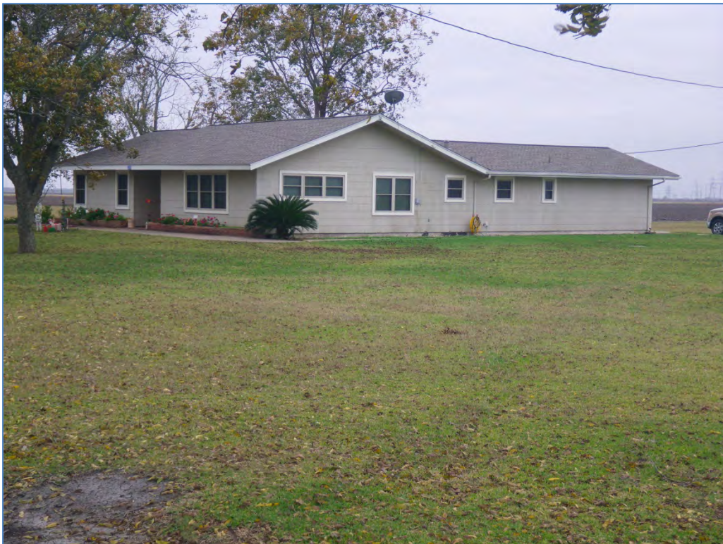
IMG1753: Looking southwest at main house, Archit-4 (12074 SR 71). (C. Borstel, Tetra Tech, December 4, 2013)
