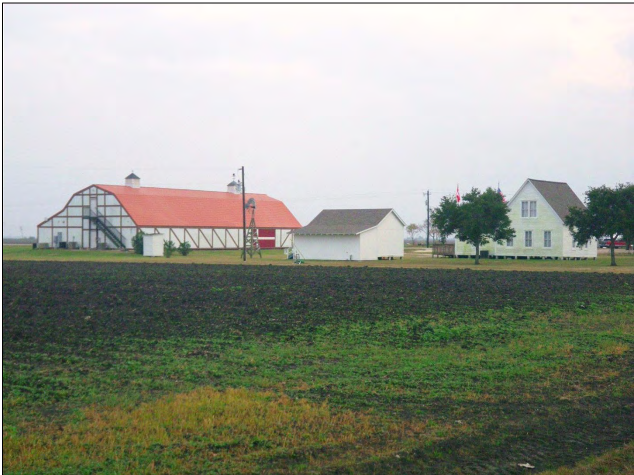
IMG1747: Looking southeast at the Danish Heritage Museum (Archit-8B, left) and the Pioneer House and adjoining buildings of the Danish settler homestead outdoor exhibit (Archit-8A, right), 153 CR 426. (C. Borstel, Ph.D., RPA, Tetra Tech, December 4, 2013)
