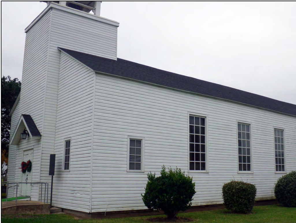
IMGP1963: Looking northwest at front and east side of Danevang Lutheran Church, showing aluminum siding and replacement windows. (C. Borstel, Tetra Tech, December 5, 2013)
