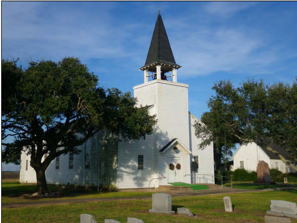
IMGP1381: Looking northeast at Danevang Lutheran Church. (C. Borstel, Tetra Tech, December 2, 2013)
