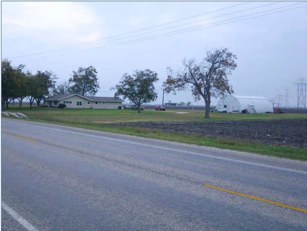
IMG1748: Looking southwest at Archit-4 (12074 SR 71). (C. Borstel, Tetra Tech, December 4, 2013)
