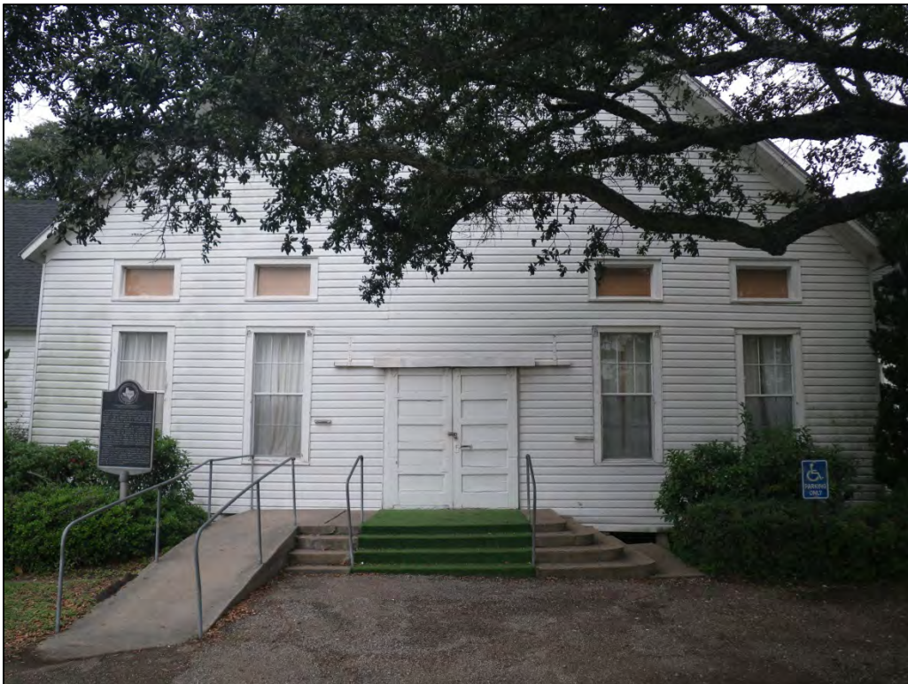
IMG1994: Looking north at front entrance of Danevang Community Hall (Forsamlingshus). Exterior is clad with aluminum siding and some windows appear to be altered. Historical marker is to left of door. (C. Borstel, Tetra Tech, December 5, 2013)
