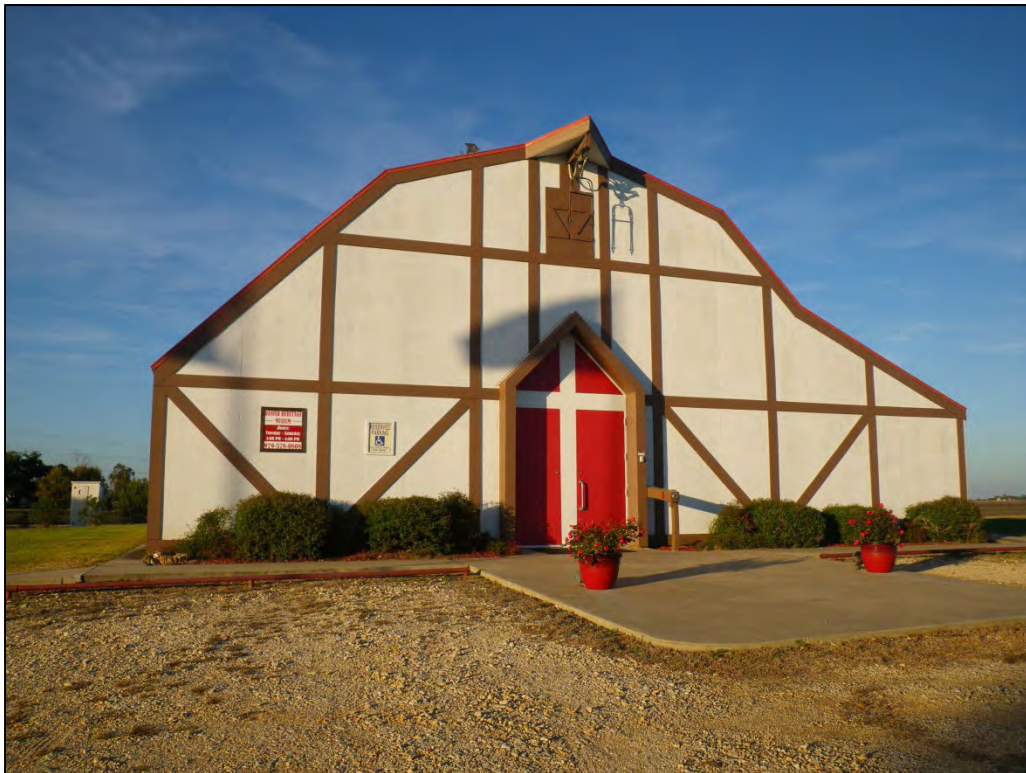
IMGP1464: Looking north at the front of the main building of the Danish Heritage Museum (Archit-8B), 153 CR 426. (C. Borstel, Tetra Tech, December 2, 2013)
