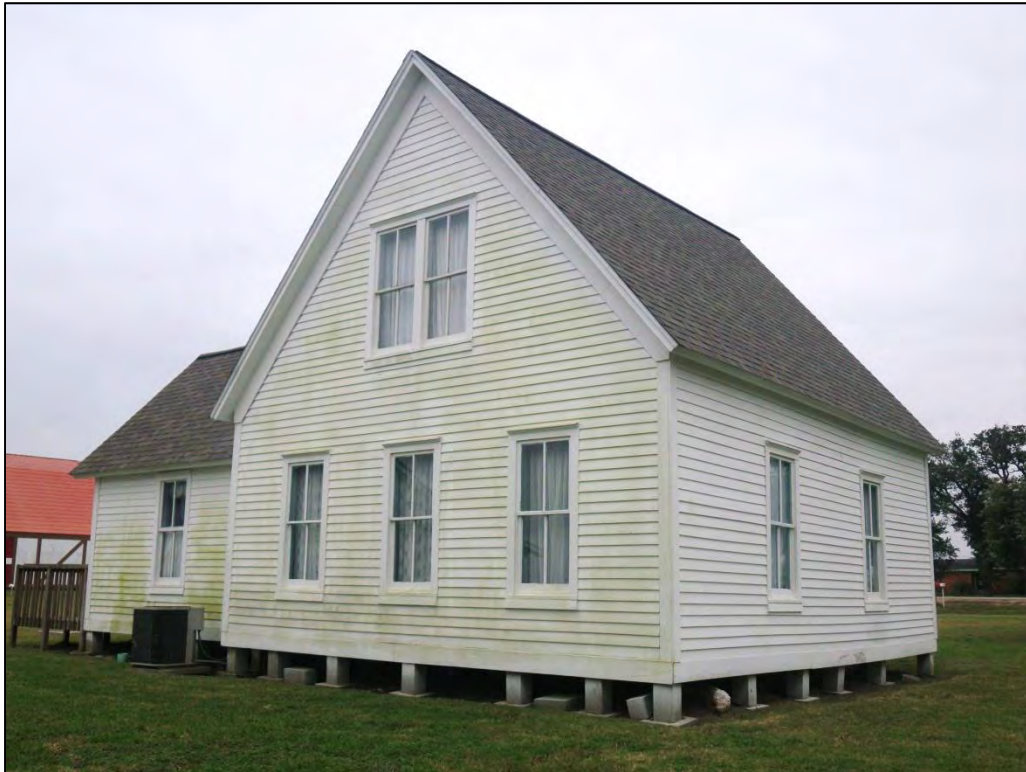
IMGP2021: Looking southeast at the Jensen House (Pioneer House), an element of Archit-8A, Danish Heritage Museum, 153 CR 426. Main house is at left; kitchen ell is at left. (C. Borstel, Tetra Tech, December 5, 2013)
