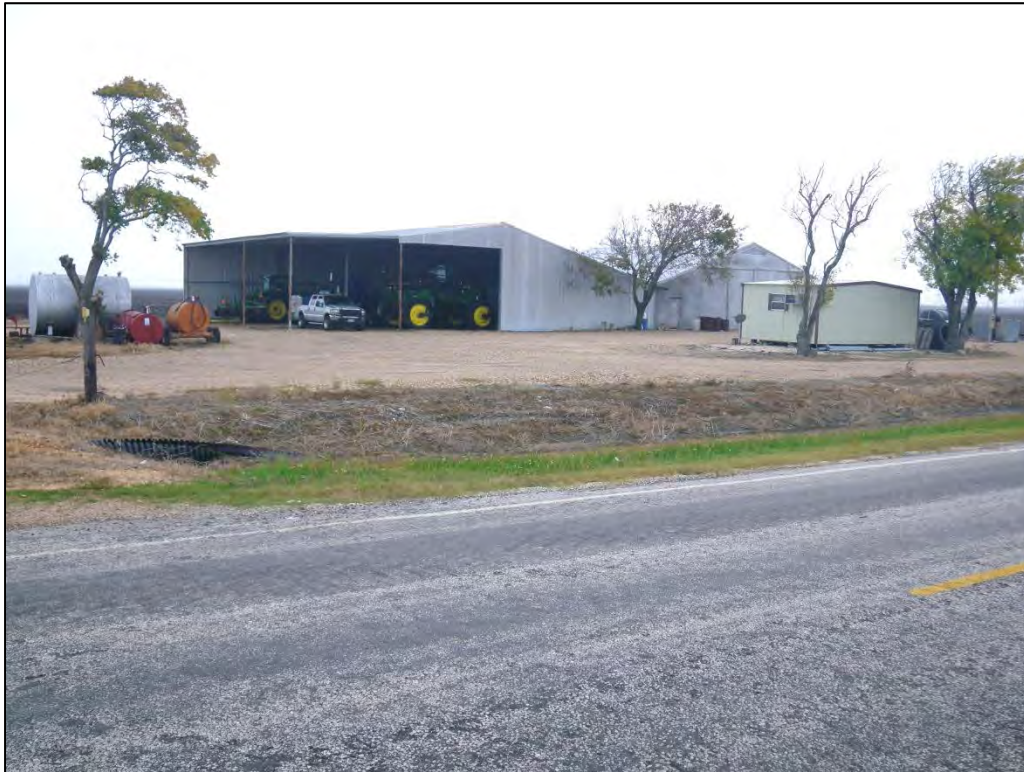
IMGP1709: Looking southwest at Archit-2 ([no number] S. FM 441). Open-bay machine shed at left constructed 1995 to 2005. (C. Borstel, Tetra Tech, December 4, 2013)
