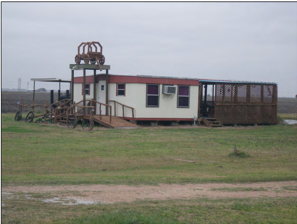
IMG1916: Looking southeast at Archit-6—portable, metal-clad, skid-mounted building used as “cabana” or office, with street address of 182 CR 426. (C. Borstel, Tetra Tech, December 5, 2013)
