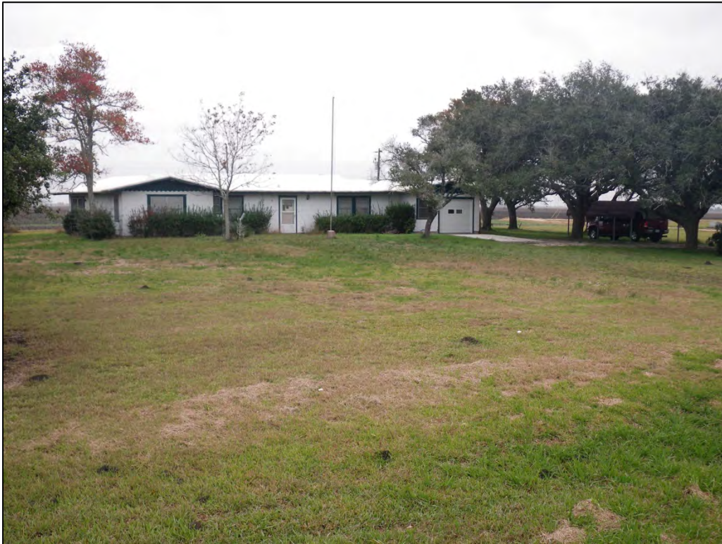
IMG1928: Looking north-northeast at Danevang Lutheran Church house or parsonage, an element of Archit-7. (C. Borstel, Tetra Tech, December 5, 2013)
