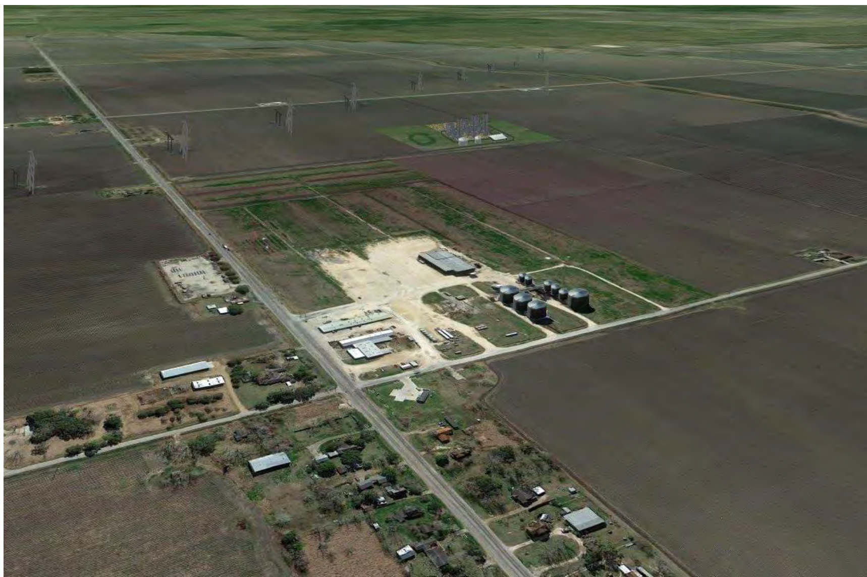
Figure 4: Aerial Overview of the Site Area from an Aerial Location to the Northeast
