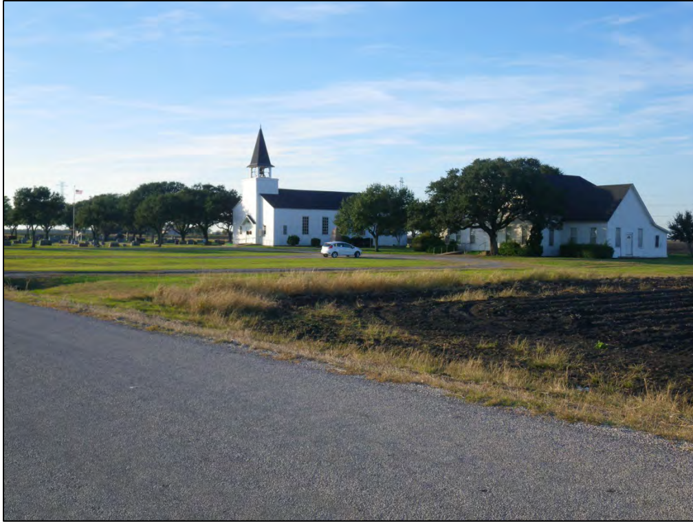
Photo 3: View northwest from CR 426 toward Danevang Lutheran Church at eastern end of surveyed area. (C. Borstel, Tetra Tech, 12/02/2013)
