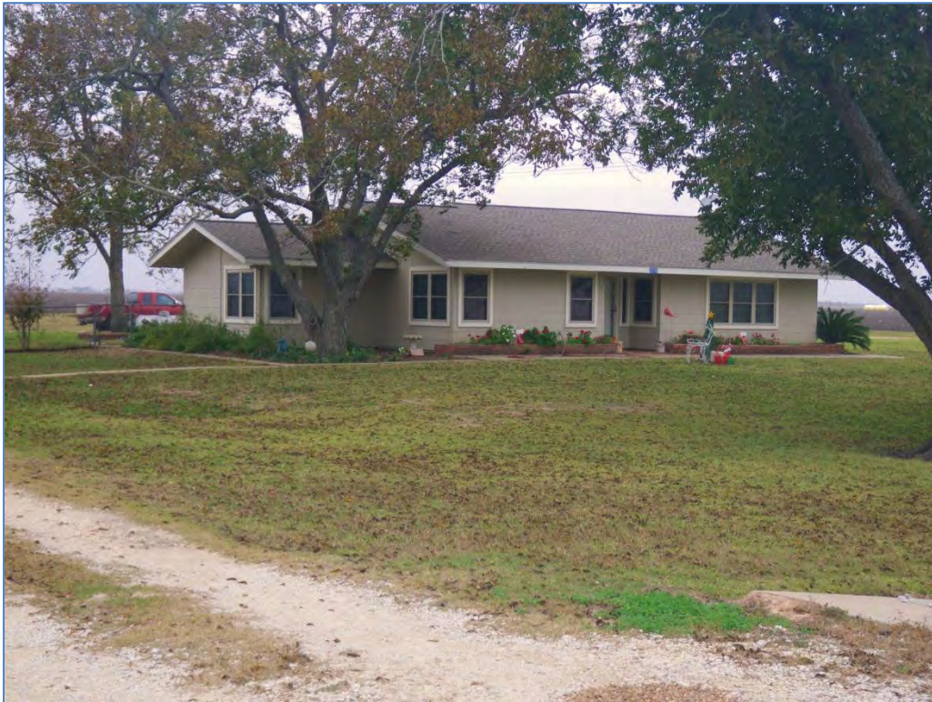
IMGP1756: Looking west at main house, Archit-4 (12074 SR 71). (C. Borstel, Tetra Tech, December 4, 2013)
