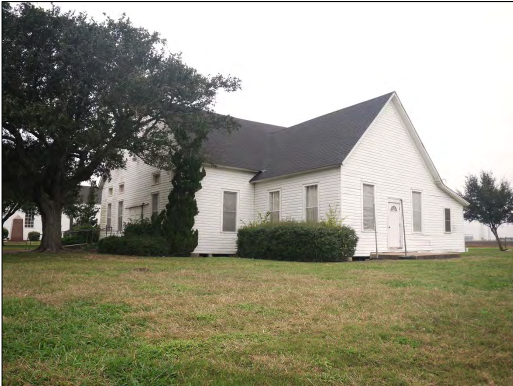
IMG2001: Looking northwest at Danevang Community Hall (Forsamlingshus) showing front (south) and east side. (C. Borstel, Tetra Tech, December 5, 2013)
