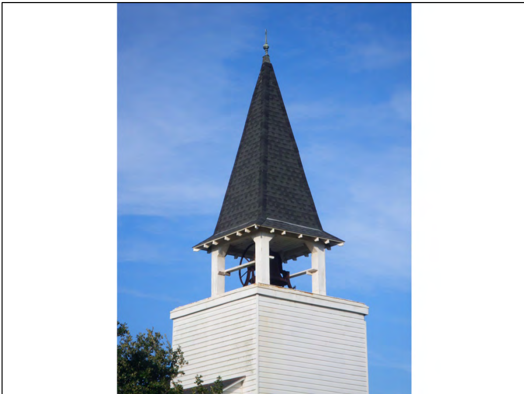
IMGP1389: Looking northeast at bell tower of Danevang Lutheran Church. Church building was relocated to this site in 1947, but tower houses bell of 1909 predecessor church. (C. Borstel, Tetra Tech, December 2, 2013)
