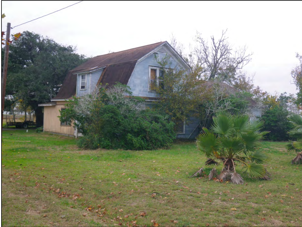
IMGP1903: Looking southeast at main house, Archit-3 (12177 SR 71). (C. Borstel, Tetra Tech, December 5, 2013)
