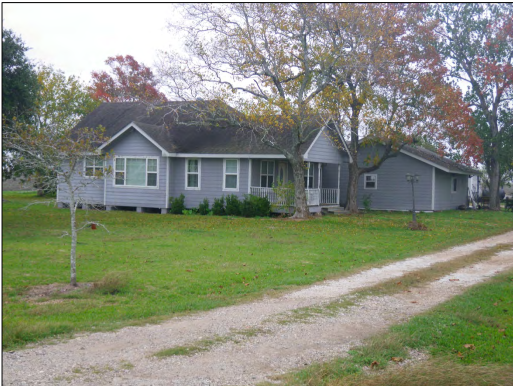
IMGP1861: Looking east at house at Archit-5 (11795 SR 71). (C. Borstel, Tetra Tech, December 5, 2013)
