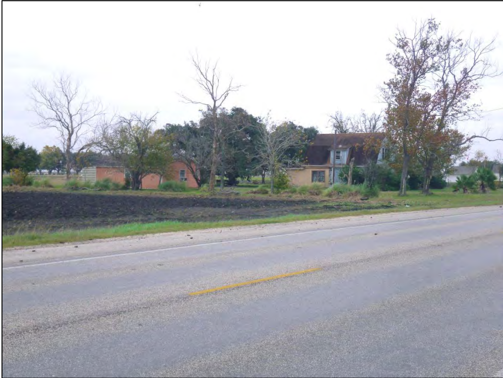
IMGP1900: Looking southeast at Archit-3 (12177 SR 71). (C. Borstel, Tetra Tech, December 5, 2013)
