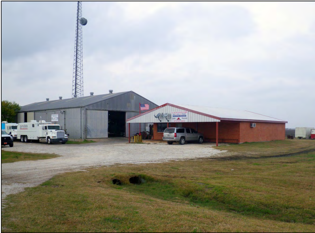
IMG1682: Looking northwest at Archit-1 (14543 S. FM 441). (C. Borstel, Tetra Tech, December 4, 2013)
