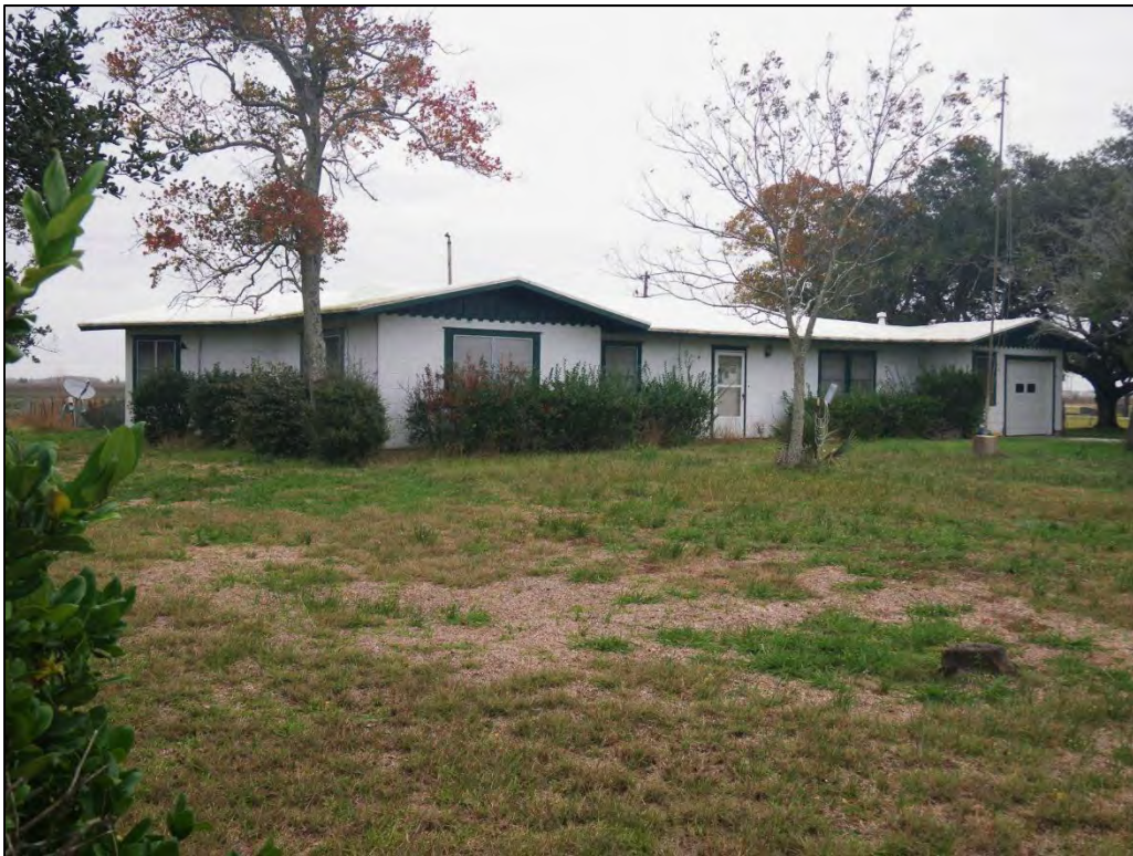
IMG1937: Looking north-northeast at Danevang Lutheran Church house or parsonage. Roof is clad with closed cell polyurethane roofing spray foam. (C. Borstel, Tetra Tech, December 5, 2013)
