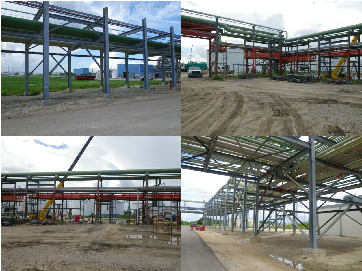
Interconnecting Pipe Racks (connect Mid Plant to West Plant), continued (Source: Whitenton Group, Inc.)
