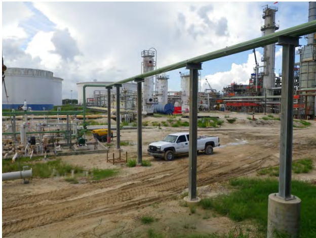
West Crude Unit (Source: Whittenton Group, Inc.)
