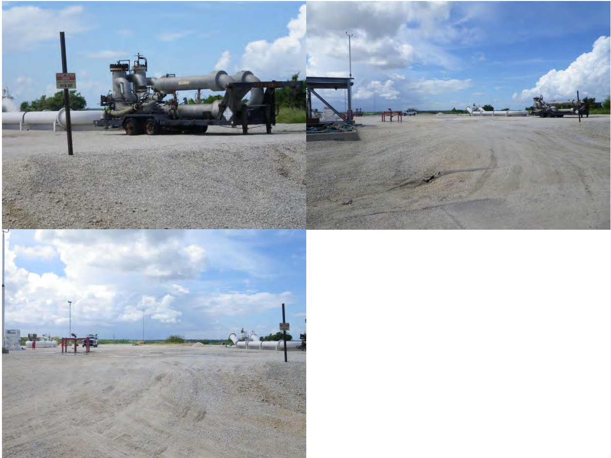
Y Grade Pipeline Pumps and Associated Equipment (new location) (Source: Whitenton Group, Inc.)
