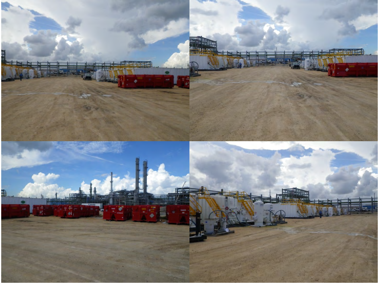
Mid Crude Laydown Area (south location) (Source: Whitenton Group, Inc.)
