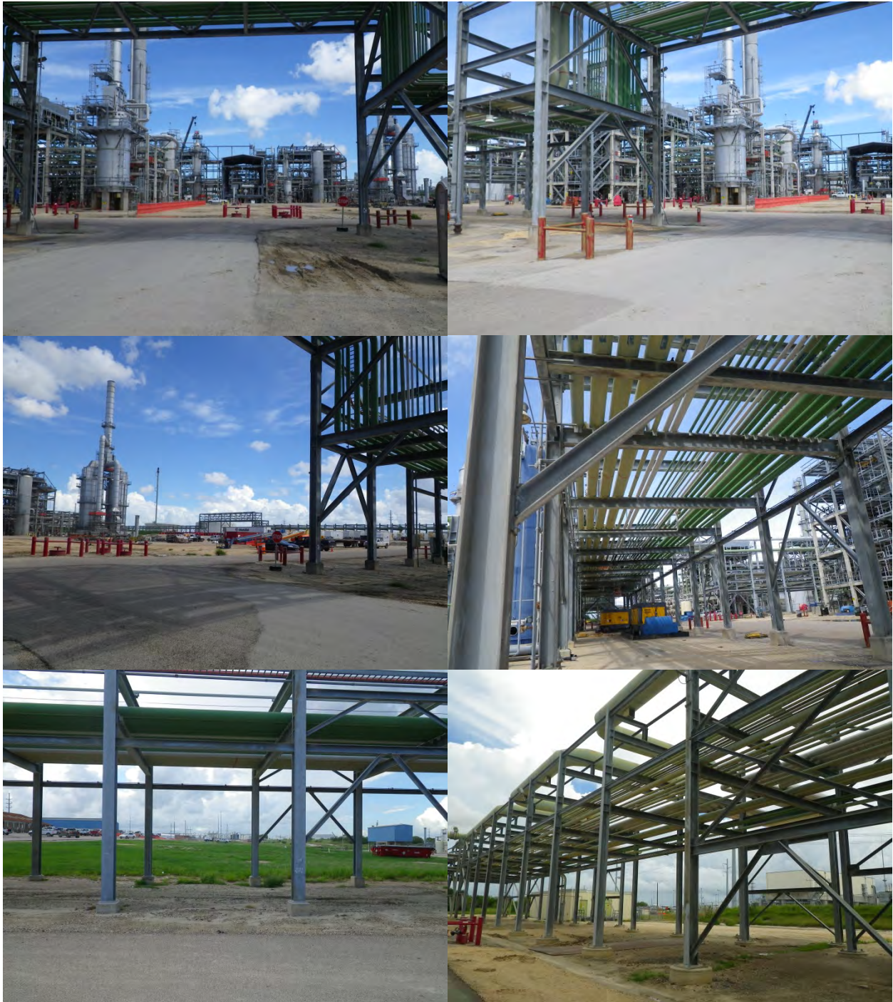
Interconnecting Pipe Racks (connect Mid Plant to West Plant) (Source: Whitenton Group, Inc.)
