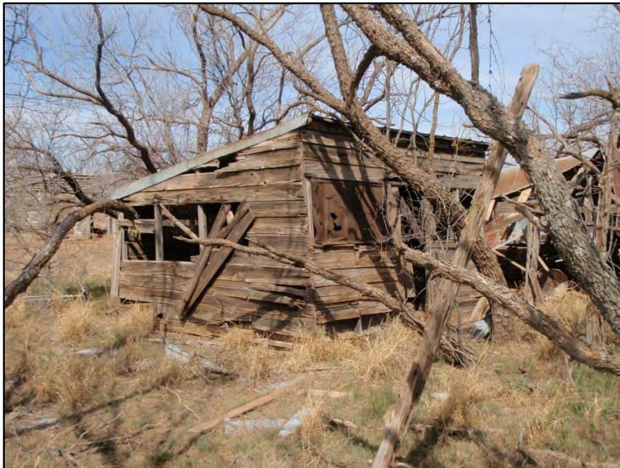
Figure 23. Resource 6 (Shed 3) front-left oblique; facing northeast.
