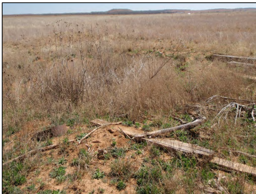
Figure 12. Dismantled oil well located in the southeast portion of the proposed project site; facing east.
