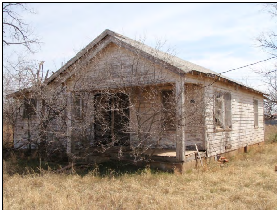
Figure 15. Resource 1 (house) front-right oblique, facing southeast.
