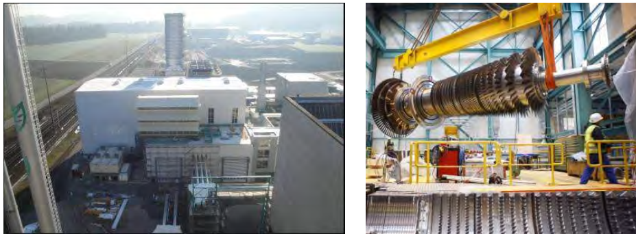
Figure 5.3: GT26 Test Power Plant
