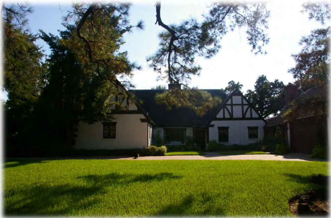
Resource 01 (5 Bay Villa): Camera facing southwest
