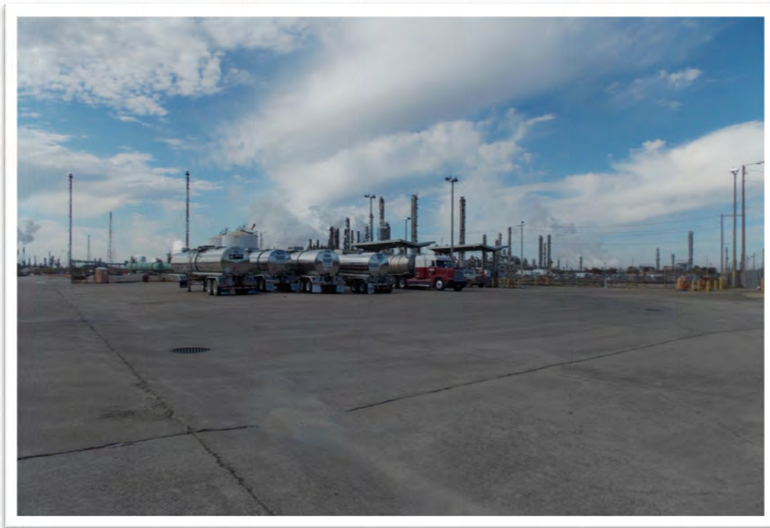
Photograph 4: Overview of Section D. Photo from northeast corner, facing southwest.
