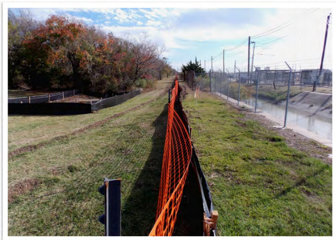
Photograph 8: Section A and C. Photo from southwest corner of Section C, facing east.
