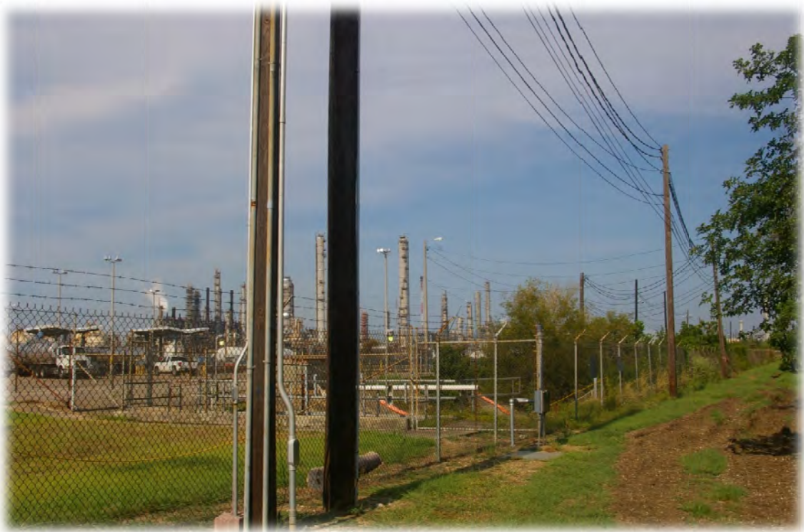
Setting View #6: View from the southern boundary of the project area, camera facing southwest
