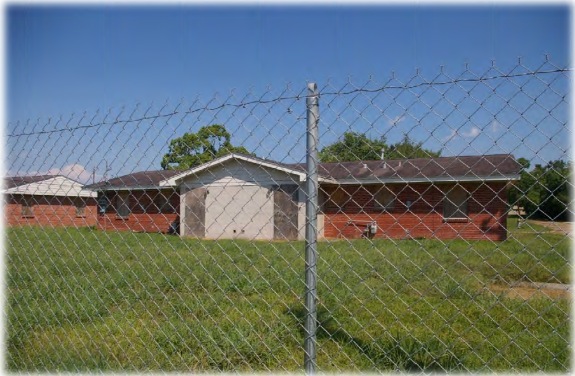
Representative view of former worker housing along Clyde Street, camera facing east
