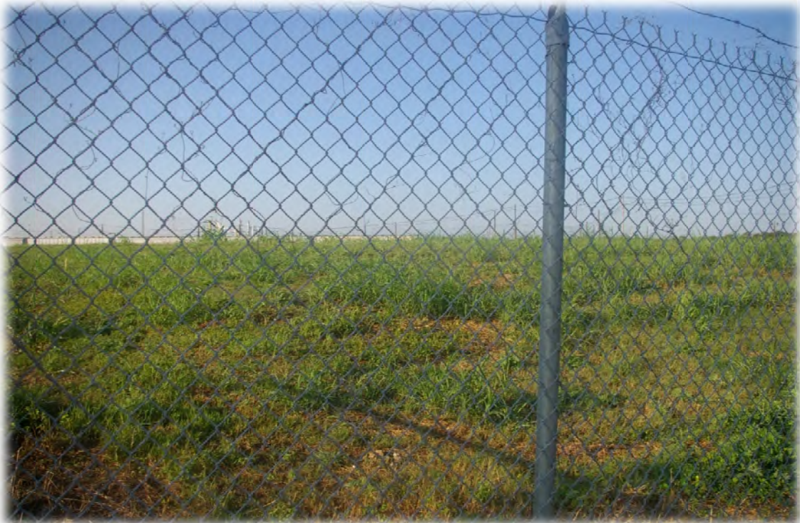
View of levee associated with historic-age canal on plant property from the public ROW, camera facing south
