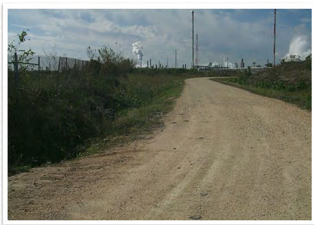
Photograph 5: Overview of Section B. Photo from bend in access road, facing southwest.
