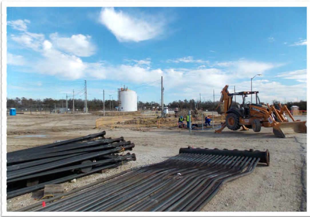
Photograph 3: Overview of Section A and D. Photo from southeast corner, facing northwest.
