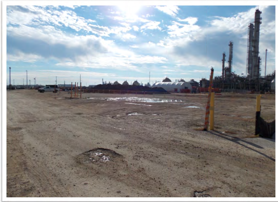
Photograph 1: Overview of Section A. Photo from northwest corner, facing southeast.
