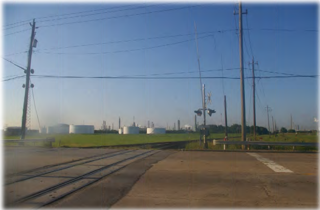
View of historic-age Missouri Pacific Railroad Grade, camera facing west
