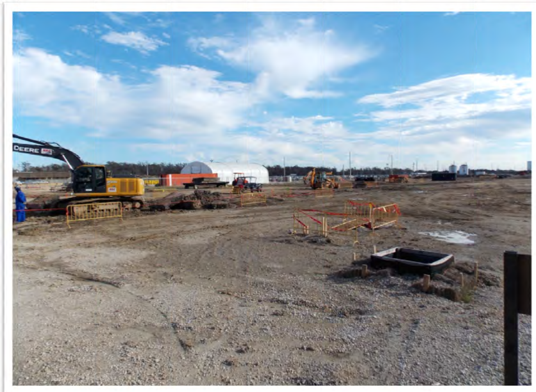
Photograph 2: Section A. Photo from southwest corner, facing northeast.
