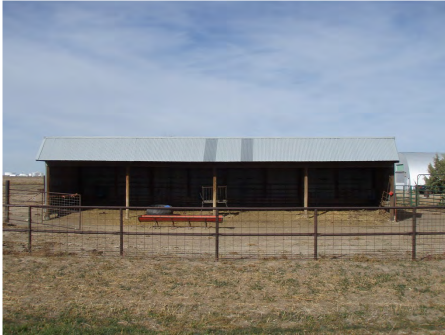
View of Resource 08B, facing north
