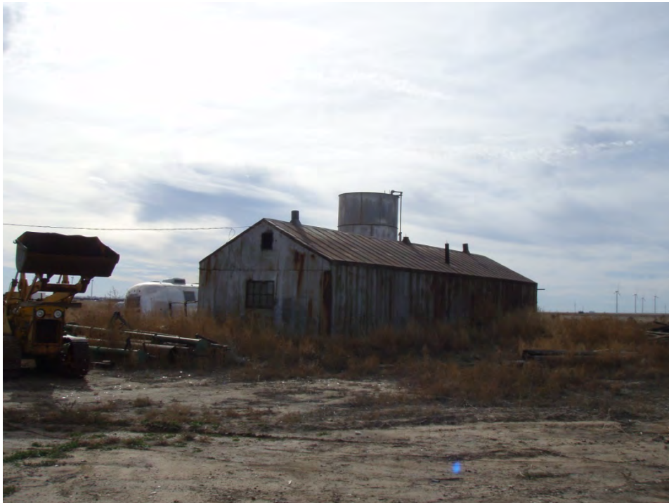
View of Resource 03C, facing northwest
