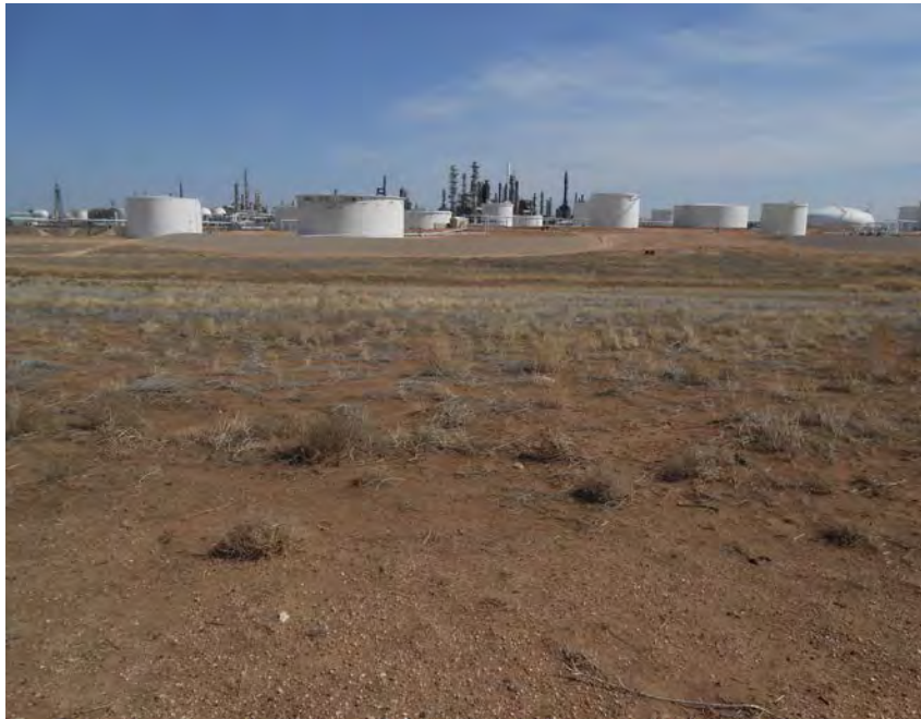
Figure 7. Overview of Tank 6 Area showing severe soil deflation caused by erosion; facing east.
