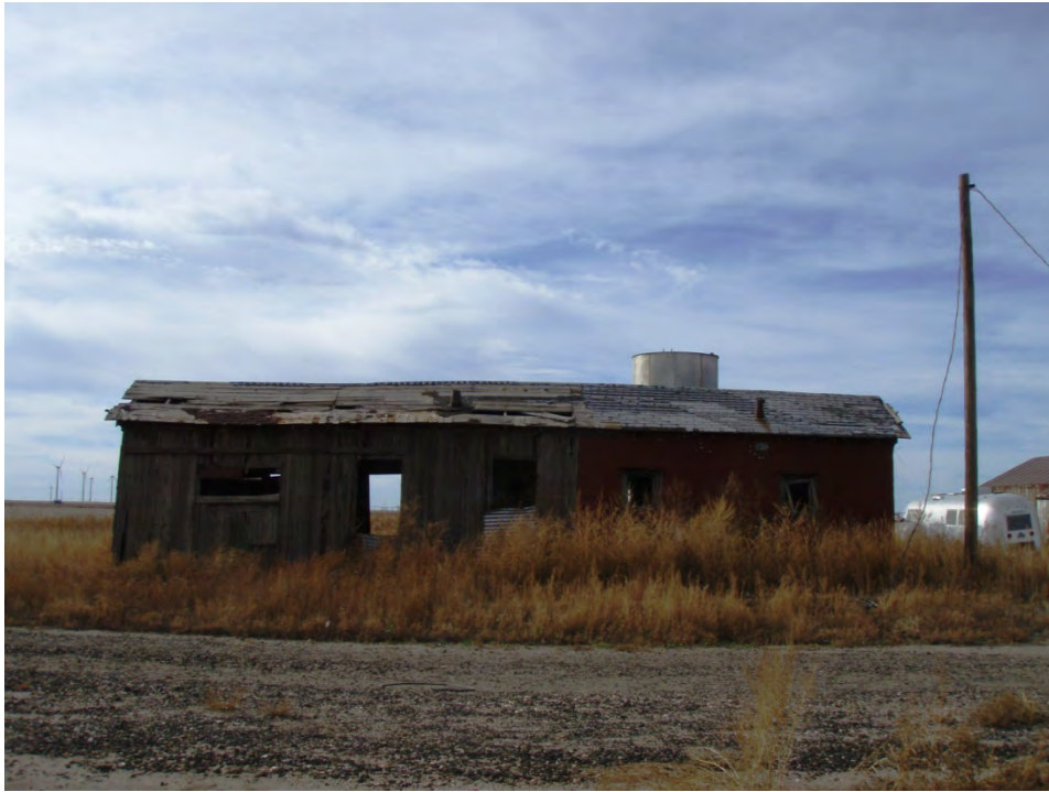
View of Resource 03A, facing west
