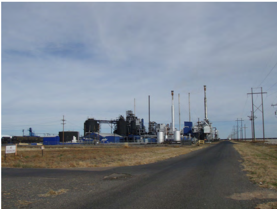
View of Resource 01 (Carbon Black Plant), facing northeast
