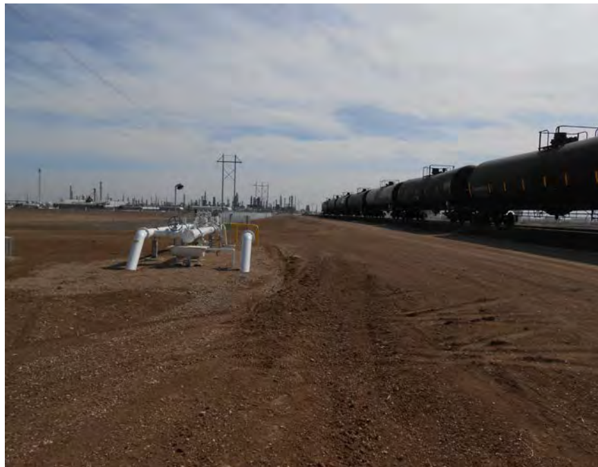
Figure 9. Overview of VTDC Area showing previously constructed railway loading area and pipelines; facing south.
