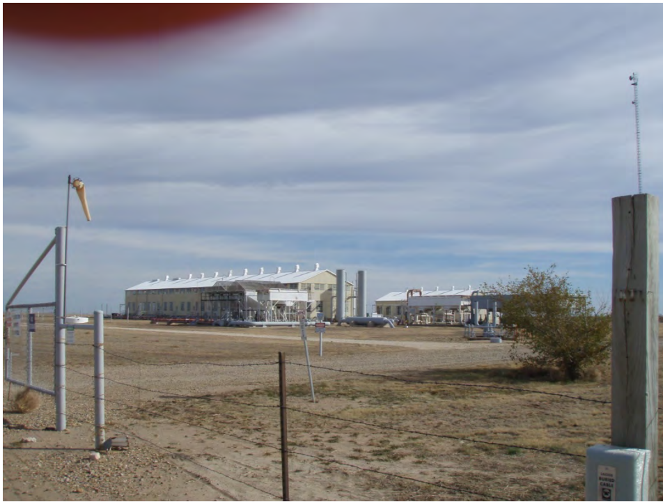
View of Resources 07A and B, facing southeast
