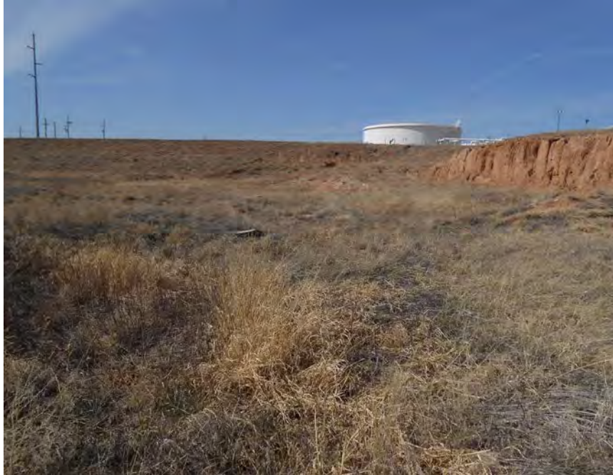
Figure 8. Overview of Tank 8 Area showing large borrow pit with steep side walls; facing northwest.
