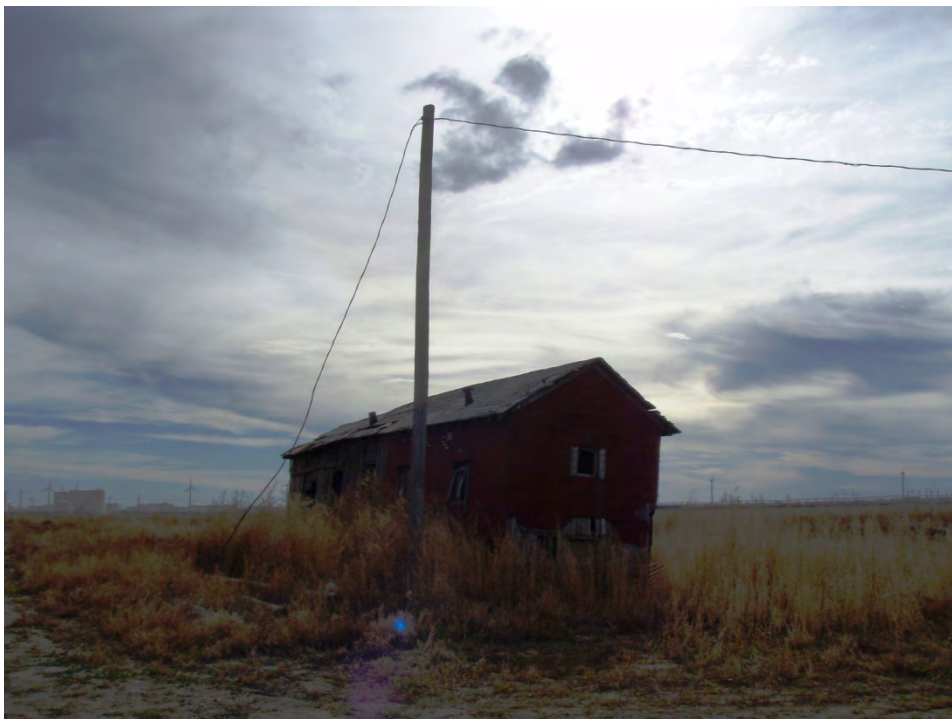
View of Resource 03A, facing southwest
