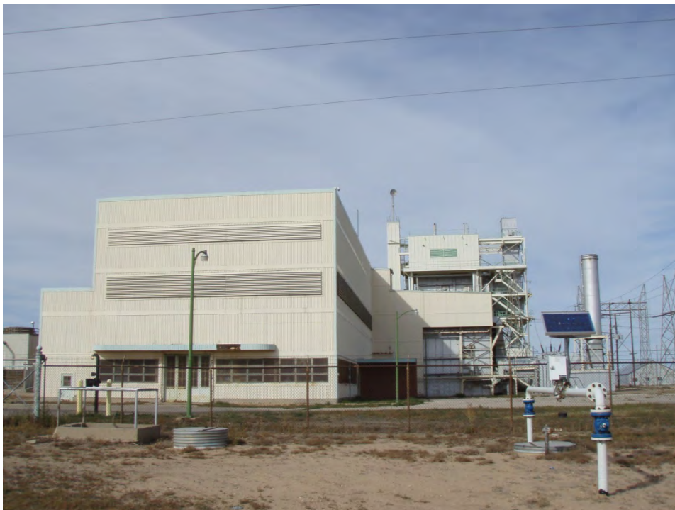
View of Resource 04 (Xcel Energy Moore County Station), facing north
