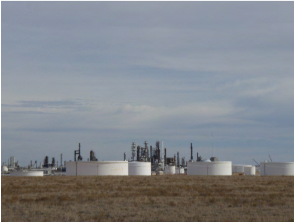
View of Resource 06 (McKee Refinery), facing southeast
