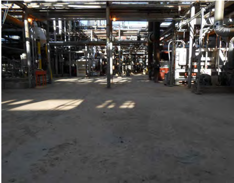
Figure 3. Overview of Nos. 1 and 2 Crude Units Area showing concrete foundation; facing west
