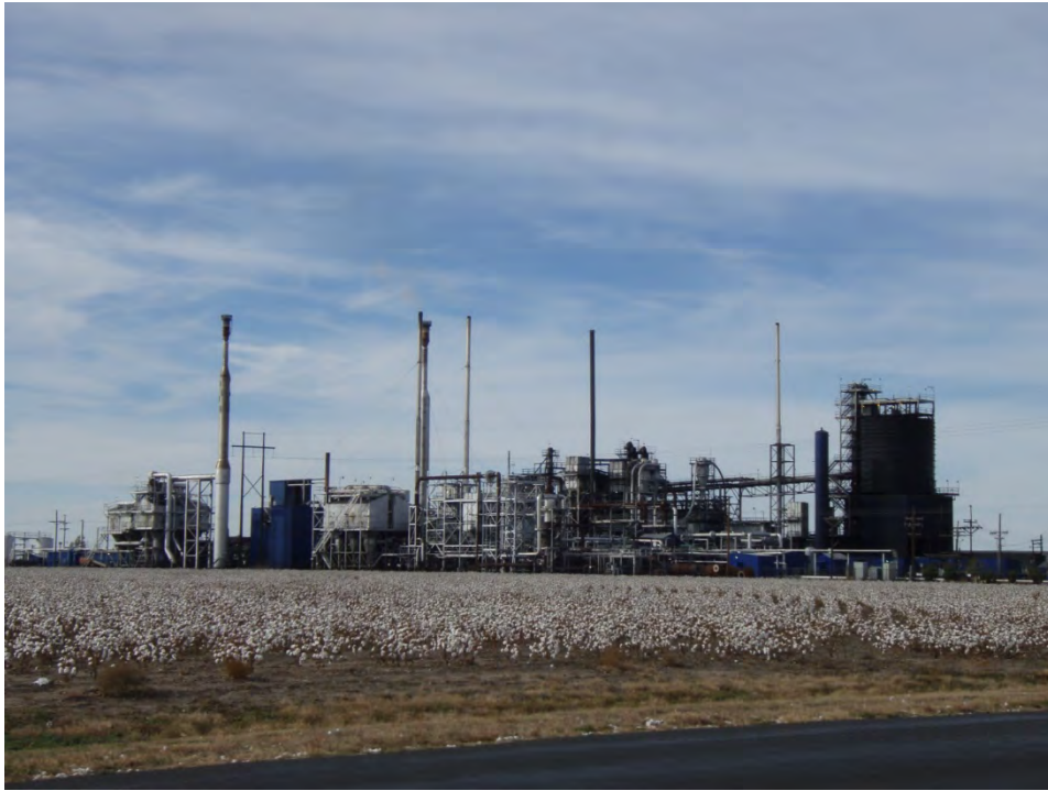
View of Resource 01 (Carbon Black Plant), facing northwest
