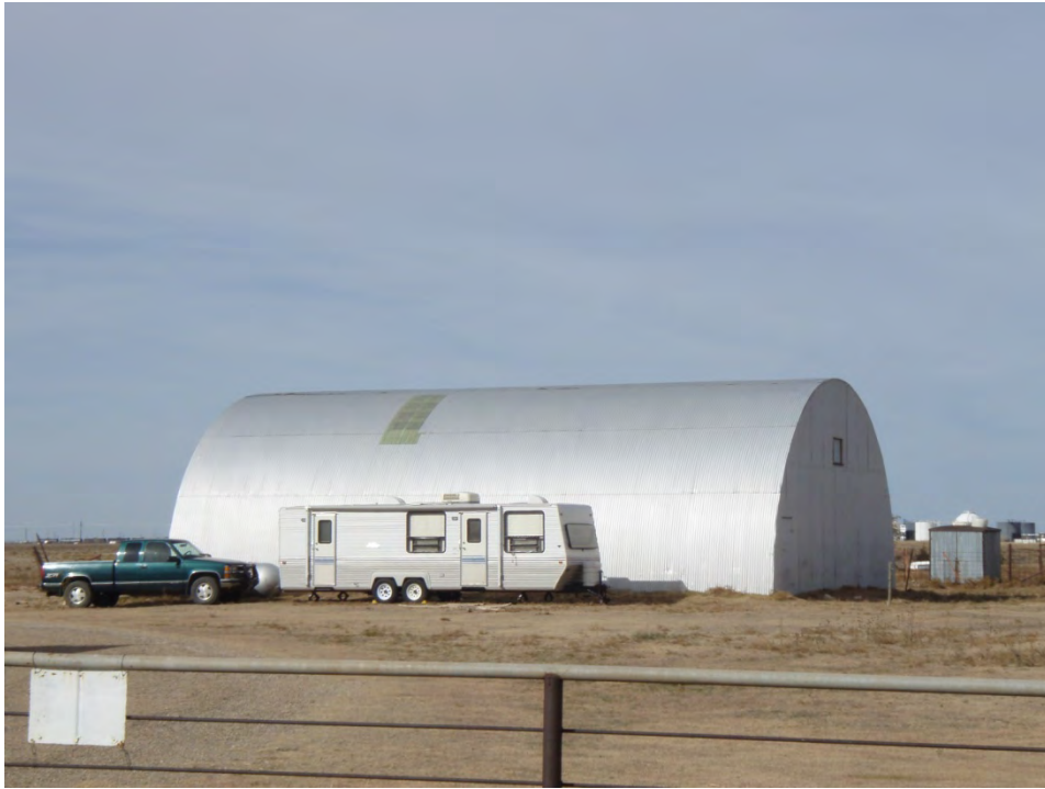
View of Resource 08A, facing northwest
