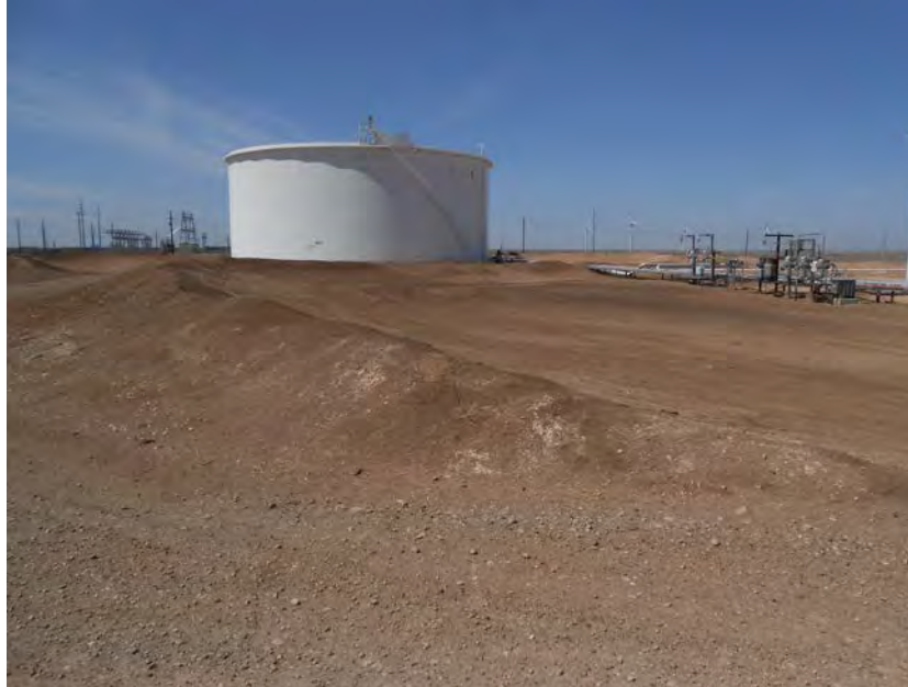
Figure 4. Overview of Tank 1 Area showing graded surface and dikes.
