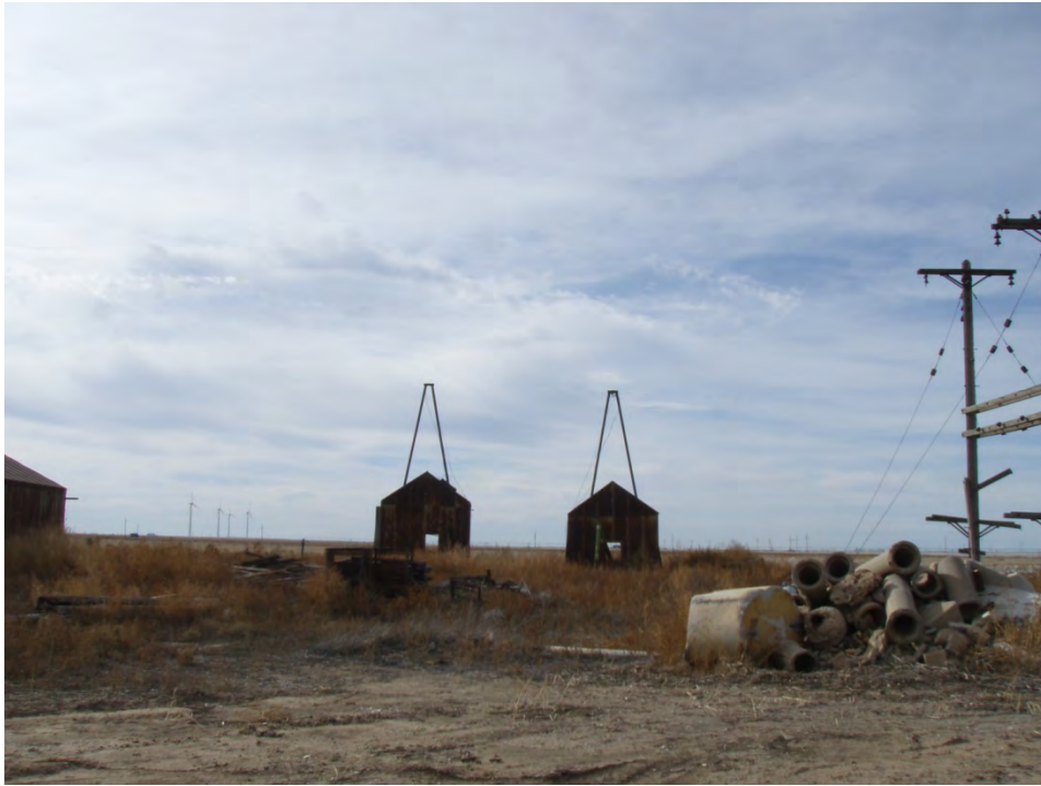
View of Resources 03D and E, facing west
