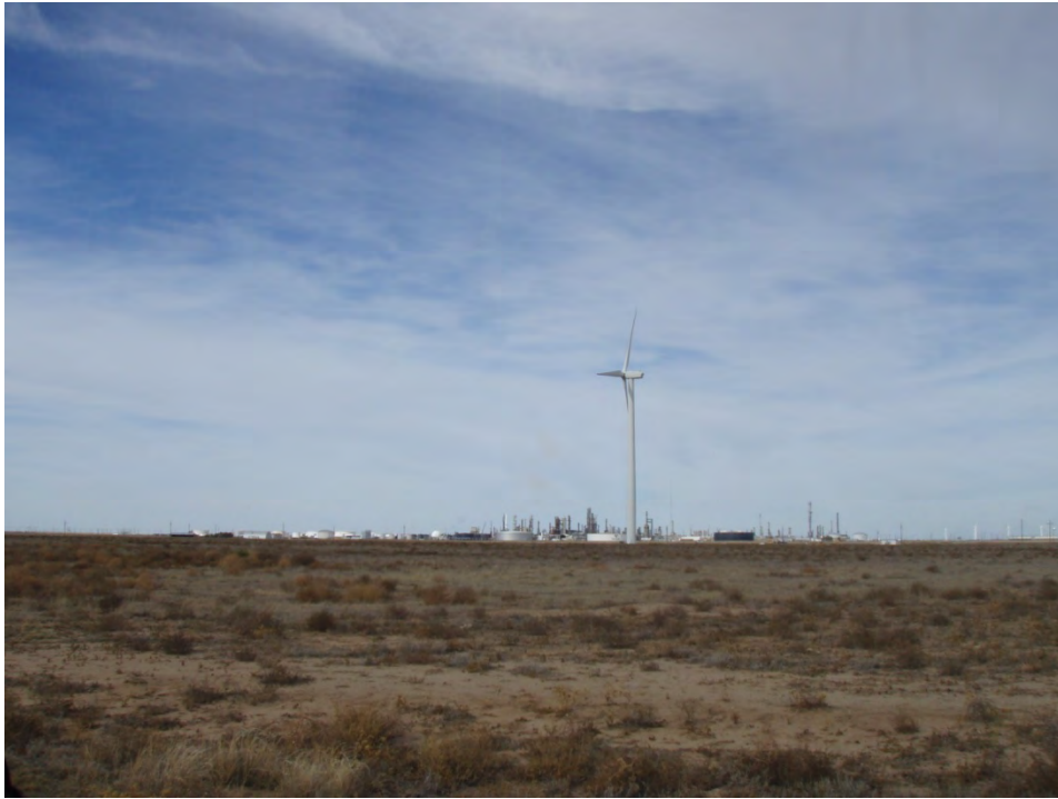
View and setting of Resource 06 (McKee Refinery), facing north
