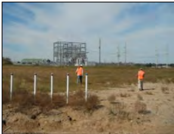
Figure 14. Survey corridor east of Highland Avenue, no shovel testing conducted.
