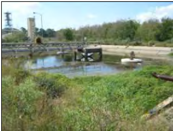
Figure 16. Area 5, wastewater treatment pond (view southwest).
