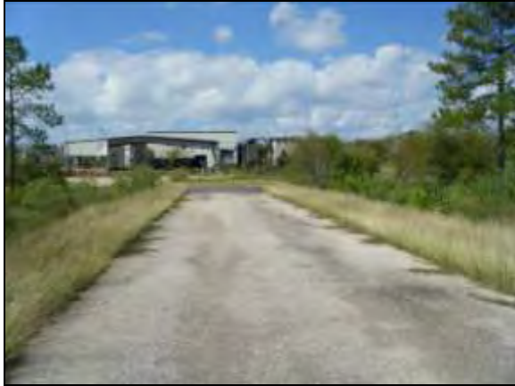
Figure 15. Area 5, overview of buildings (view west).
