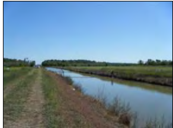
Figure 5. Irrigation canal in Area 2 (view east).
