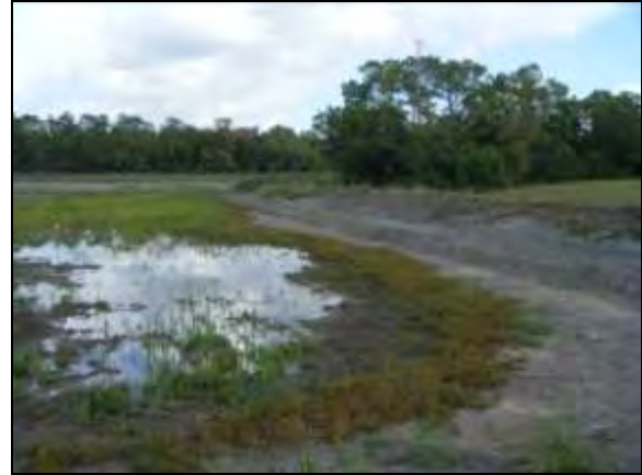
Figure 13. Area 4, detention basin (view north).
