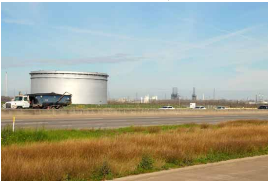
Photo 16 Petroleum tanks and old field
