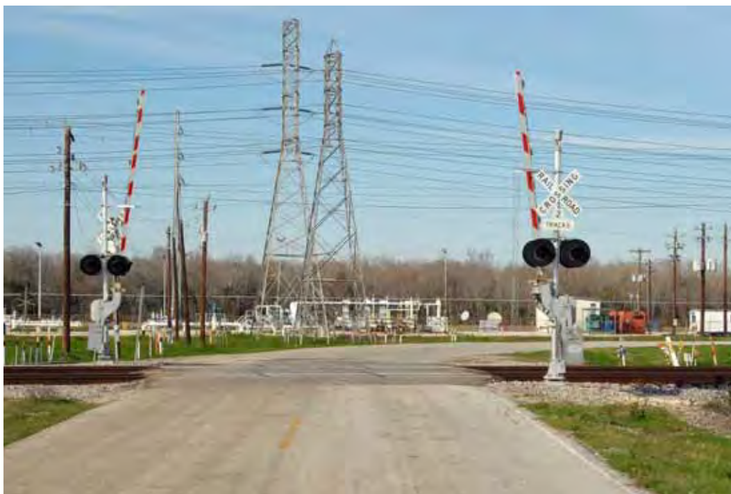
Photo 19 Maintained/mowed ROW in foreground with dense woods in background
