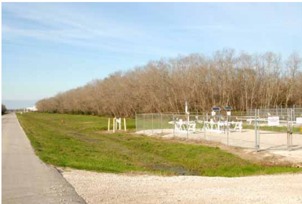
Photo 21 Maintained/mowed ROW in foreground with dense woods in background
