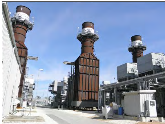
PHOTO 1: SHEC PLANT SITE
