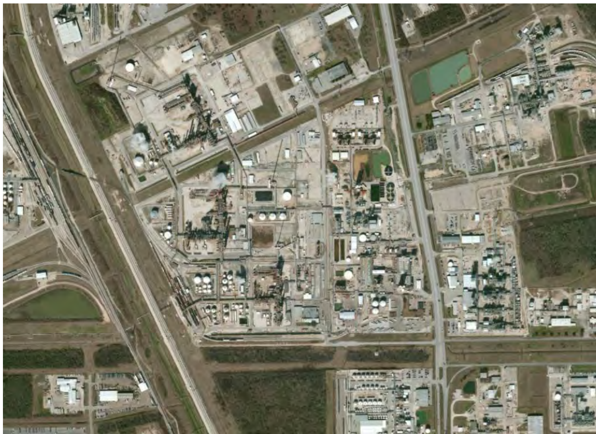
Figure 1: Location of the Air Liquide Large Industries U.S., LP Plant
