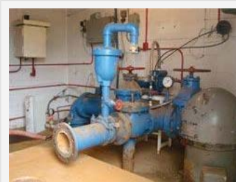
The pump that the Village of Crestwood used to draw water from an underground aquifer, which was used to supplement their drinking water drawn from Lake Michigan. This picture was taken after the pump was already disconnected from the well and taken out of service.
