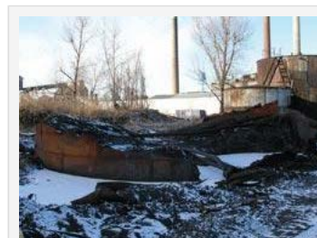
Storage tank that was dismantled for scrap metal and released coal tar sludge material that tested positive for benzene
